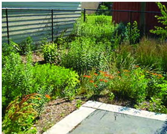
Image 36: Rain gardens should be planted up with native plants that thrive with occasional overflow from a water butt
