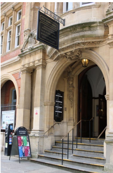
Entrance to the Old Town Hall which houses the Reference Library and Museum of Richmond
