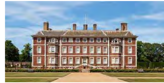
4 Ham House was completed in 1610. It is Grade I listed with a mix of early Jacobean English Renaissance and classical style architecture.
