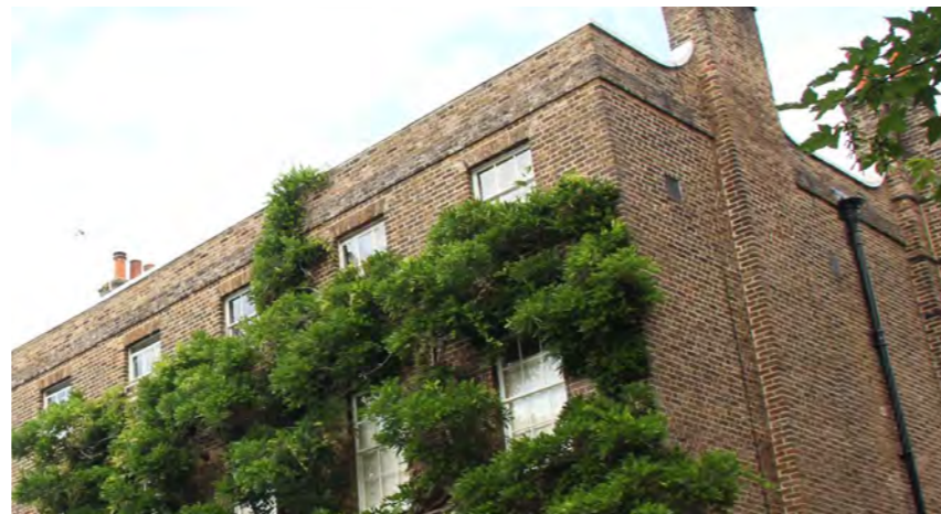
Langham House (Rear) - Grade II Listed Building
