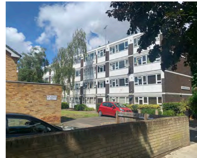
Sutherland House and Scott House
