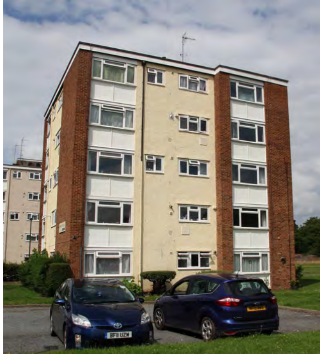
5 storey block with parking court in foreground
