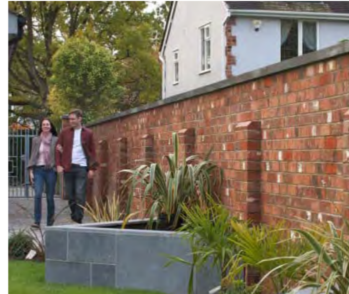
Traditional brick wall with piers and coping
