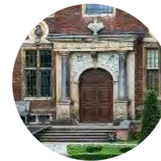
Ham House Strong entrance emphasised through change in material and detailing.
