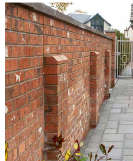
Typical brick wall - Western boundary & rear gardens
