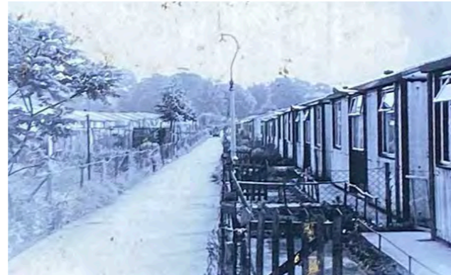
View down Woodville Road towards Beaufort House.
