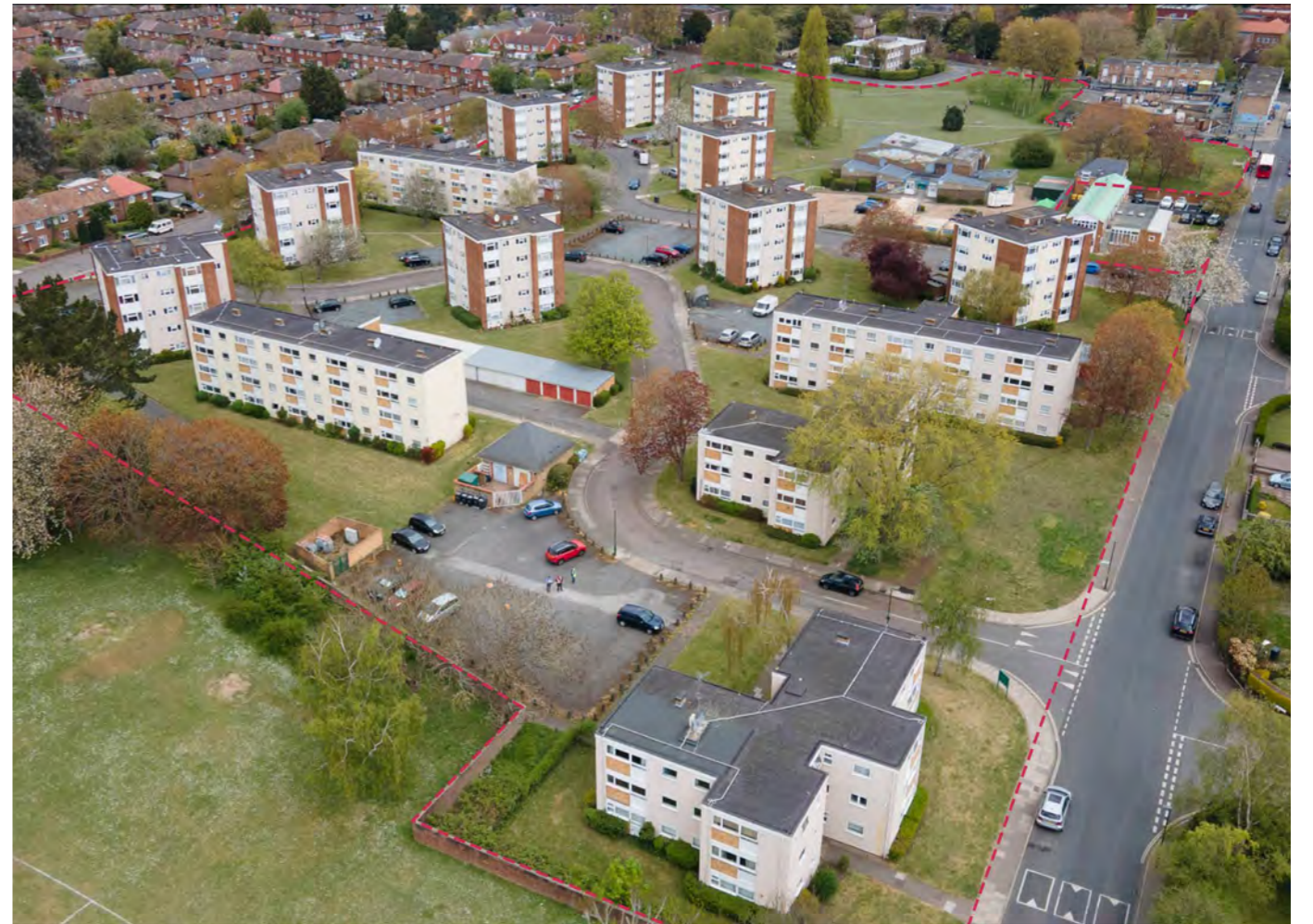
Aerial view looking east from the south west corner of the site
