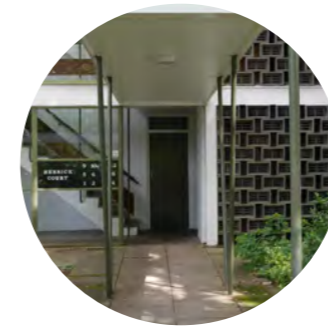
Parkleys Estate Canopy and column supports highlight entrance into building.
