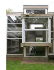
Langham House Close - James Stirling Vertical circulation and horizontal banding
