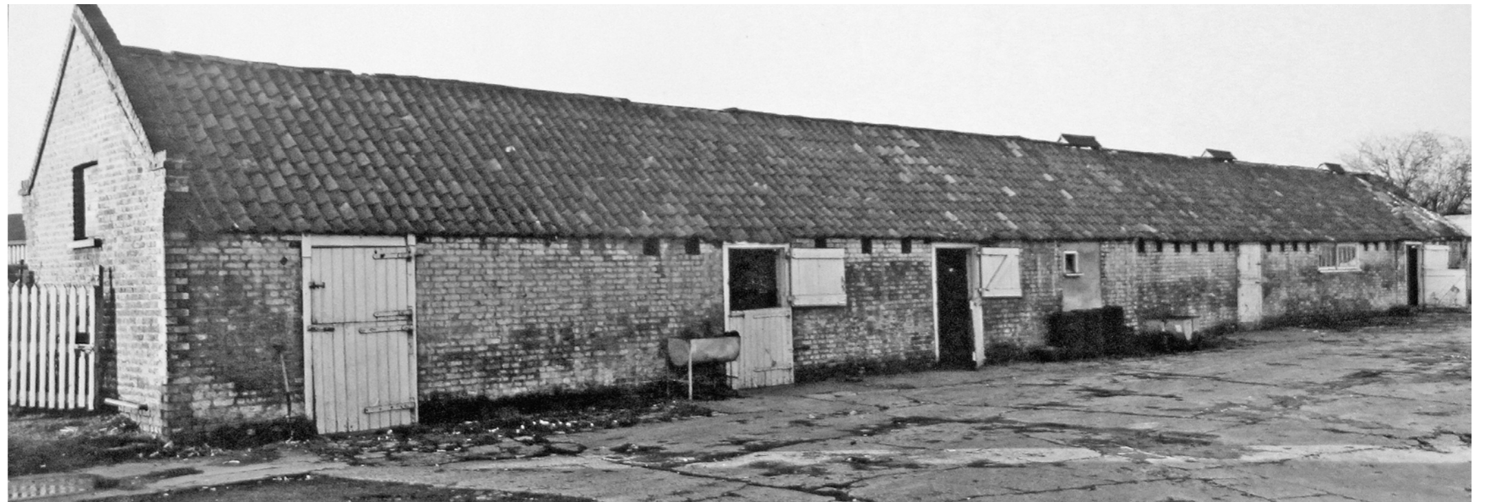
Barn Structures on Manor Farm - Now Demolished
