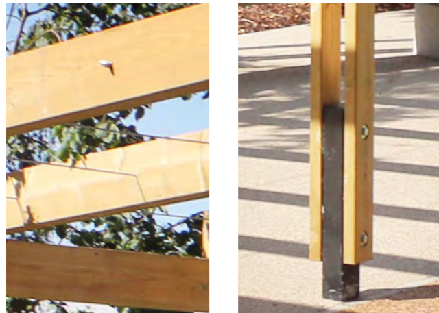
Slatted timber structure and metal shoe detailing
