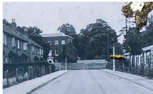
View down Woodville Road towards Beaufort House.
