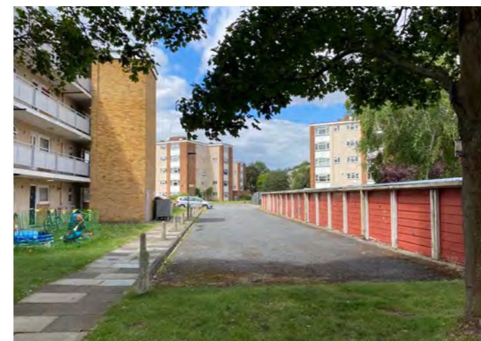
Garages and access close to Grieg House
