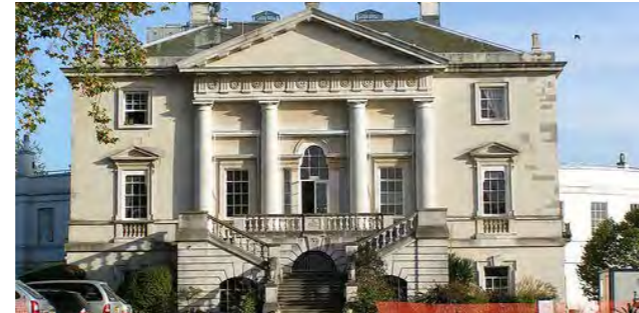
7 White Lodge was completed in 1730 for King George II. Originally called Stone Lodge, the name New Lodge was given to distinguish it from Old Lodge and later the name White Lodge was given. It now houses the Royal Ballet School. (Grade I listed).
