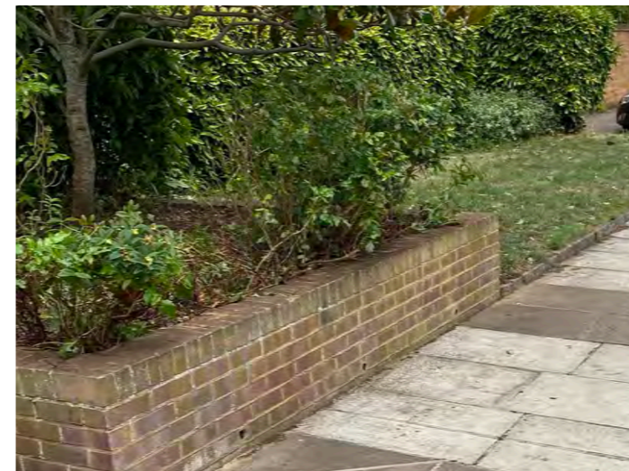
Raised planters to reinforce corners
