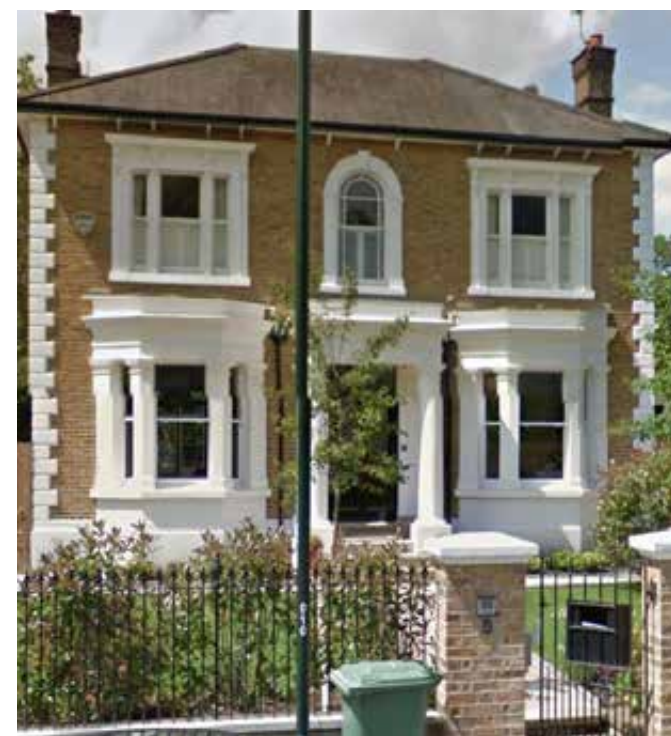
Iron Railings, Ailsa Road
