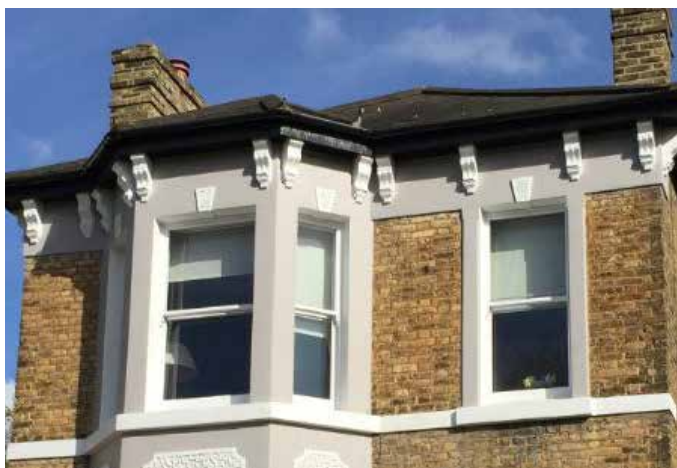
Timber sash in a Victorian house
