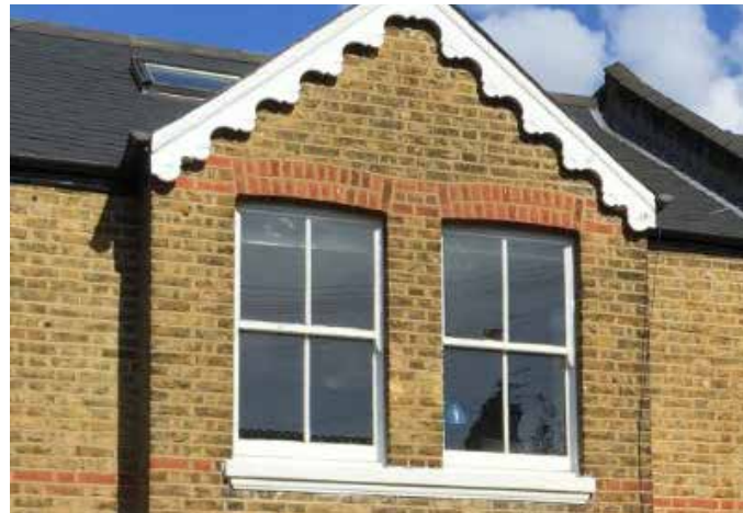
Timber sash in a Victorian house
