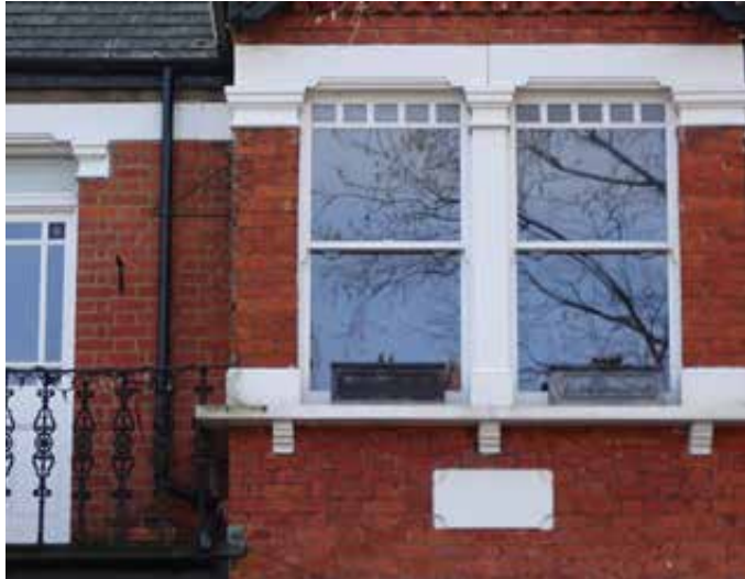
Timber sash with decorative glazing bars in a c. 1900 house
