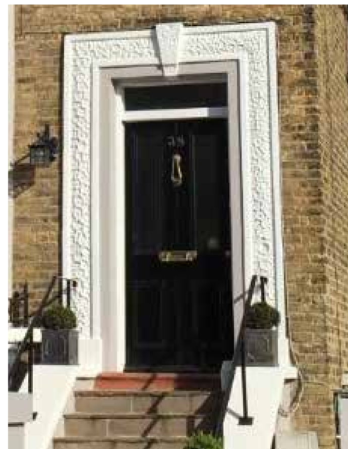
Four panelled timber door with rectangular fanlight in a Victorian house
