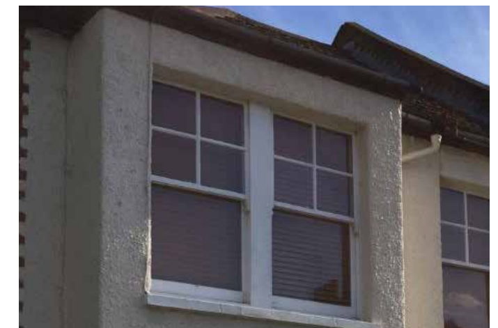
Timber sash windows in a house from the early twentieth century
