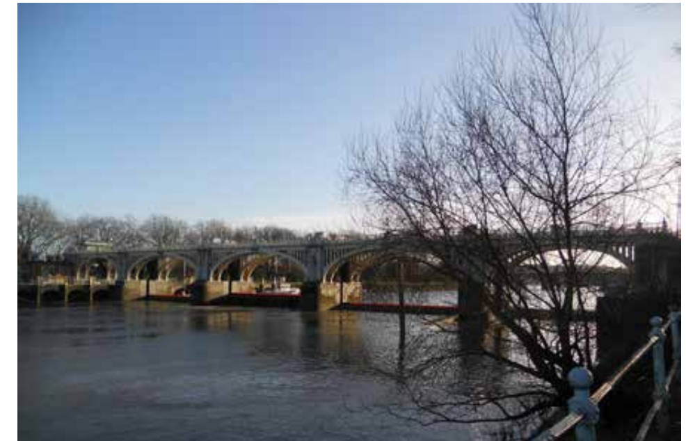
Richmond Footbridge, Lock and Sluices
