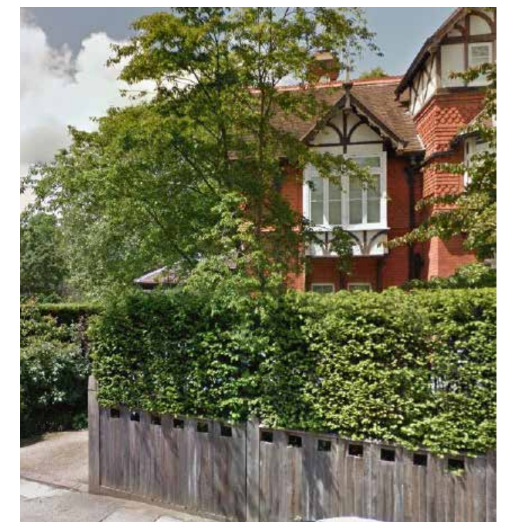
Fencing, St Margarets Road
