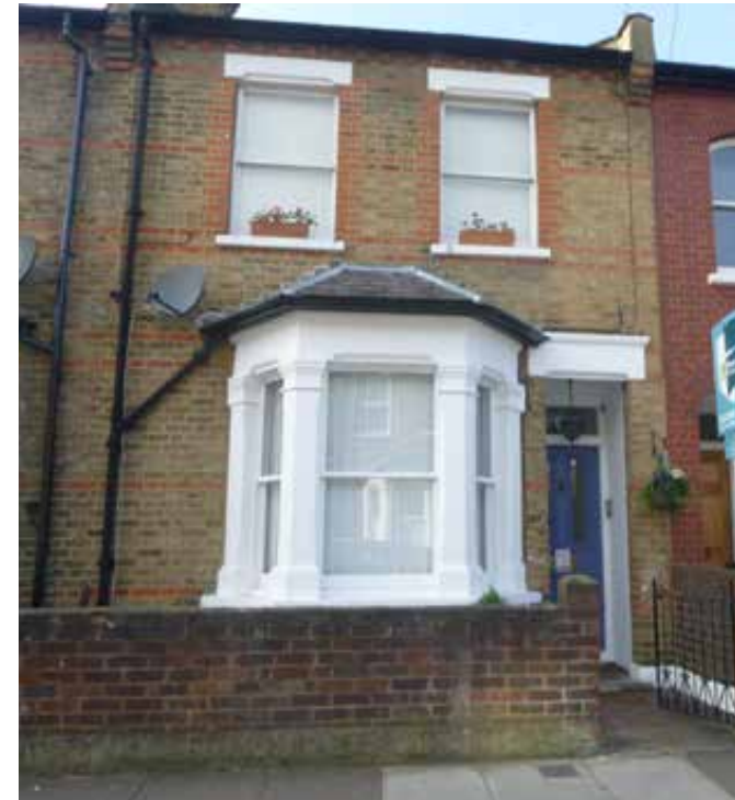
Boundary wall, Haliburton Road
