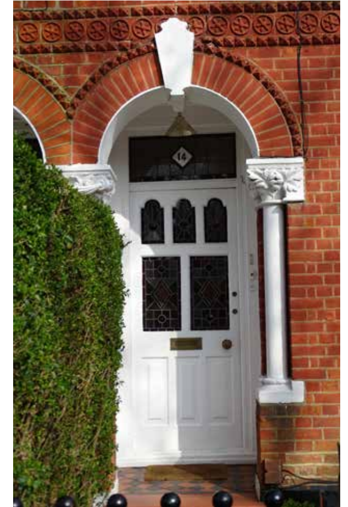
Timber panelled door, in a late Victorian / early Edwardian house
