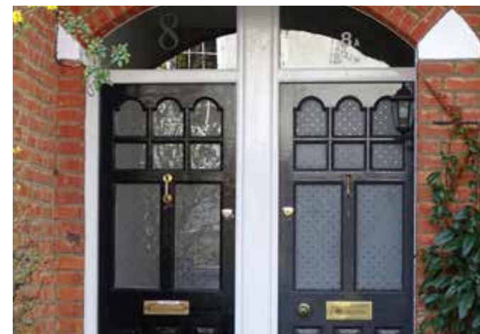
Timber panelled door with decorative lights in a c. 1900 house
