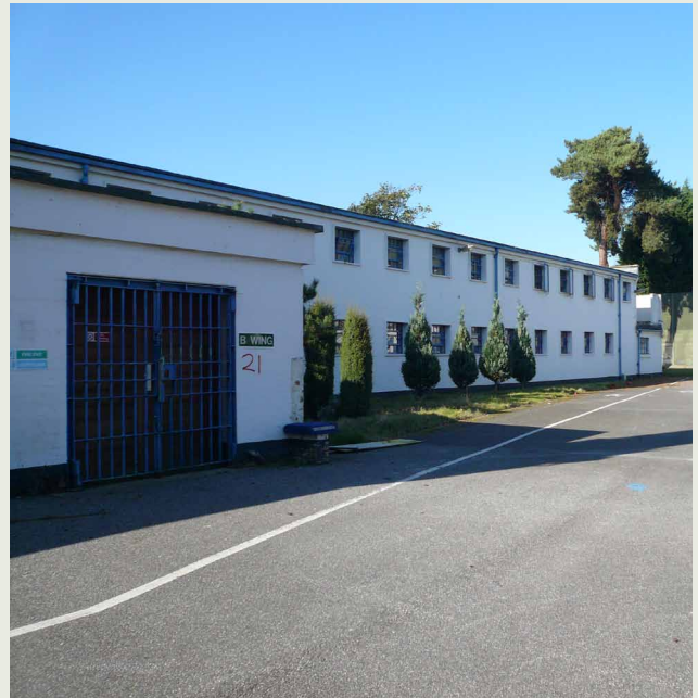
View south from inside the site
