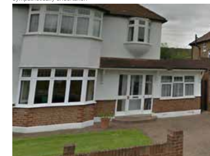
The adaptation to this property has used matching bricks and maintained the brick plinth with render above. The front boundary wall is in keeping.
