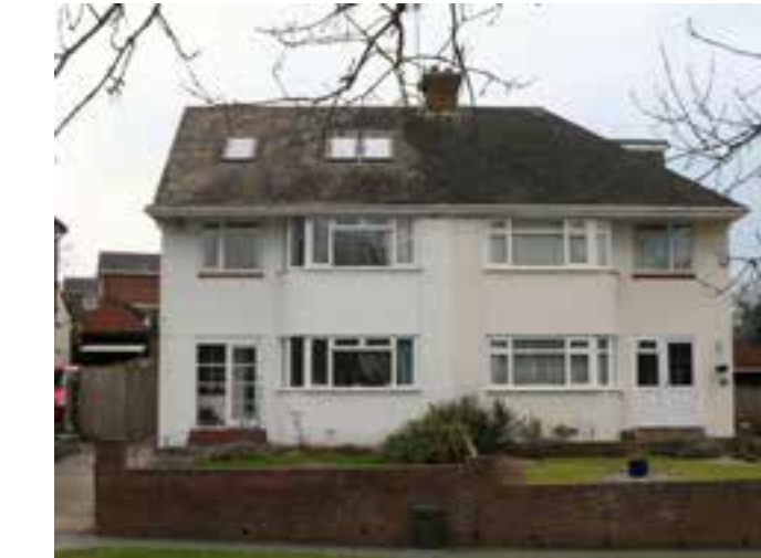
Don't extend your house with development that is dominating or out of scale. Try and retain roof lines and shape (e.g. by keeping a pitch roof)
