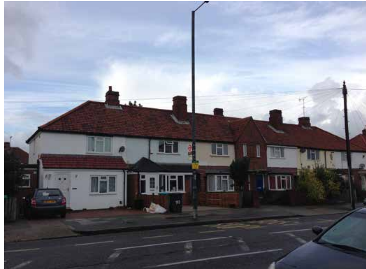
Hospital Bridge Road
