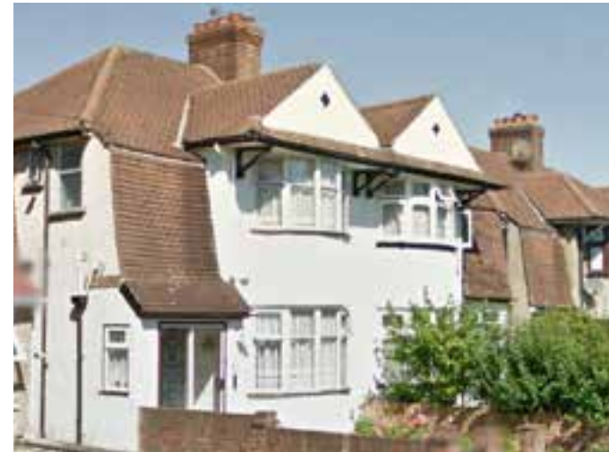
Arts and Crafts style, multiple pitched roofs, tile detail on a pitched gable, bow window. This pair of adjoining properties have white painted render
