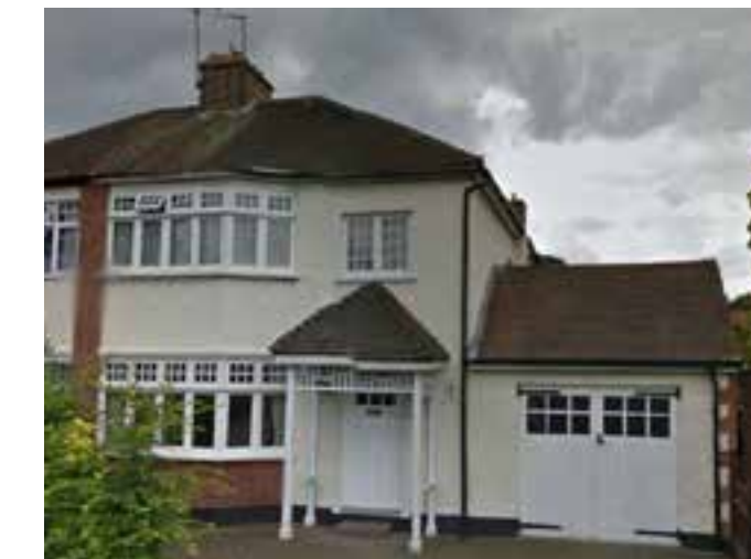
A garage extension, replacement windows and restoration work have been sympathetically undertaken
