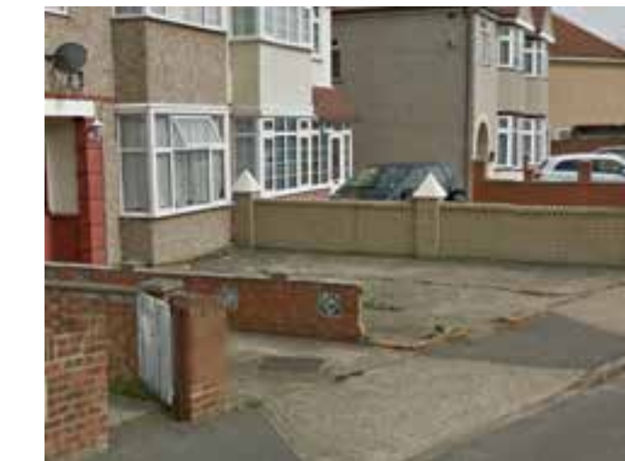
Don't remove boundary walls at the front of your house. If replacing or maintaining boundaries try to match the brick with your house.
