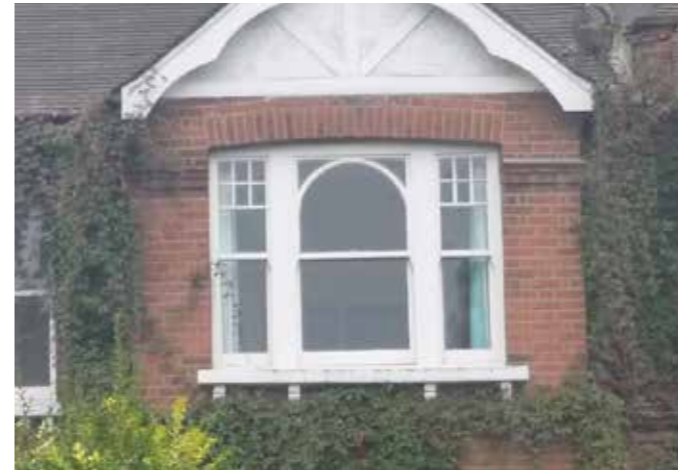
Edwardian sash windows with arch motif in the upper pane, and narrow margin hybrid sashes to either side, set in a simple brick reveal
