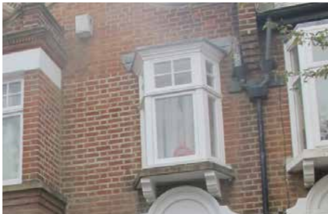
Edwardian timber oriel window with casement opening
