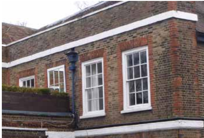
Georgian six-over-six sash windows, set flush with the façade in rectangular brick reveals
