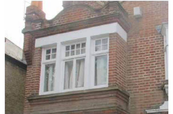
Edwardian Queen Anne-style timber casement windows with a multi-pane transom light, set in a projecting square bay
