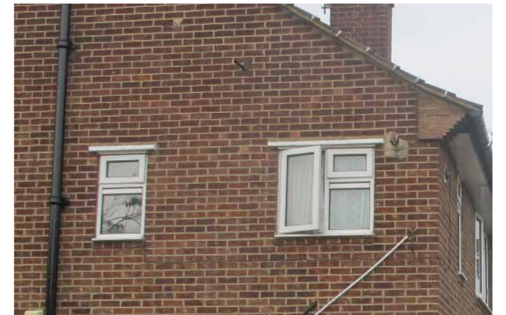
Post-war uPVC windows with different casement openings
