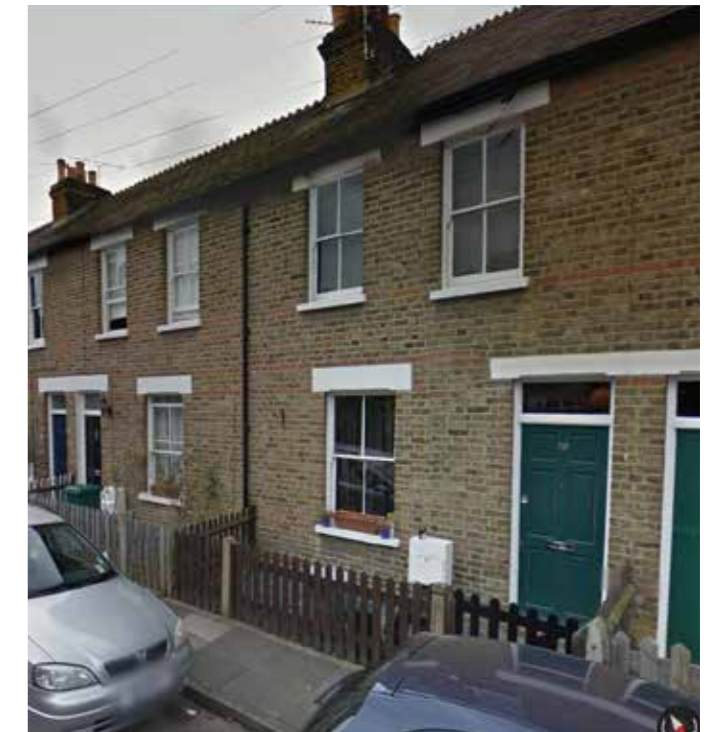
Fencing - Victoria Road
