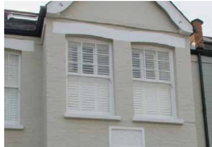
Edwardian hybrid sash windows in a square bay, the upper sash containing nine regular lights
