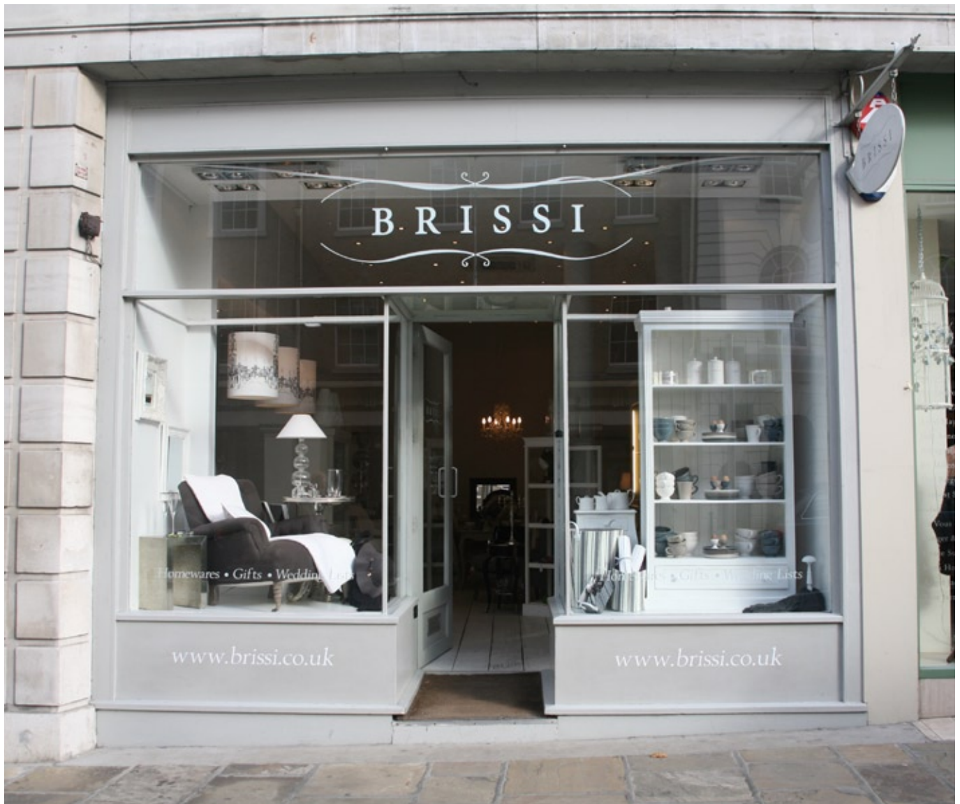
Modern signage integrated with a traditional shopfront design
