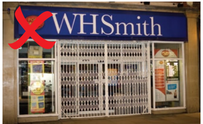
External security shutters appear less integrated
