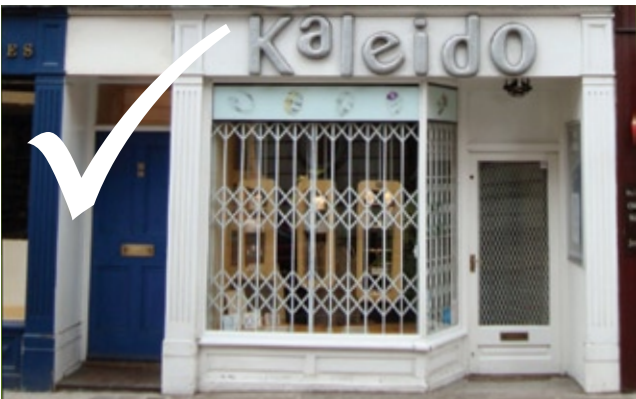
Internal shutters that have been successfully integrated with the character and design of the shopfront
