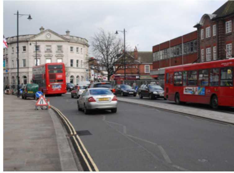
View along King St. with the Water Lane entrance to the right hand side
