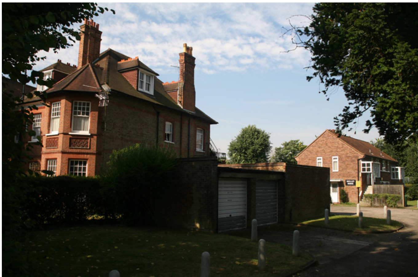
Single-storey flat-roofed garage blocks adjacent to No 34, Strawberry Hill Road
