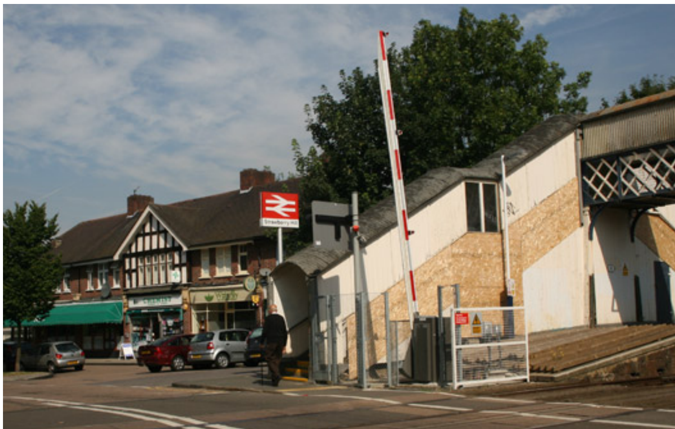
Rear view of station approach from the end of Strawberry Hill Road
