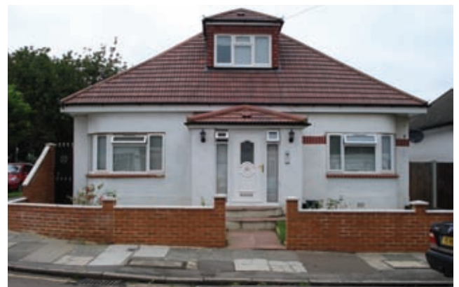
5. Inappropriate alterations – brick wall, porch (size and style), front dormer, roof tiles, fenestration, chimney removed, brick bands on façade mostly painted over.
