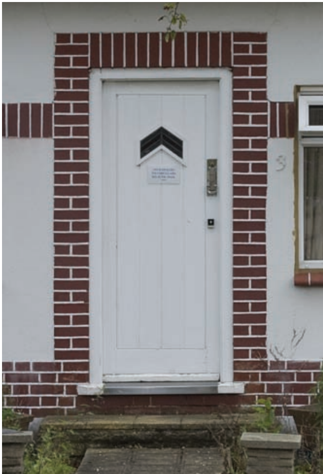
7. Original detail – original door
