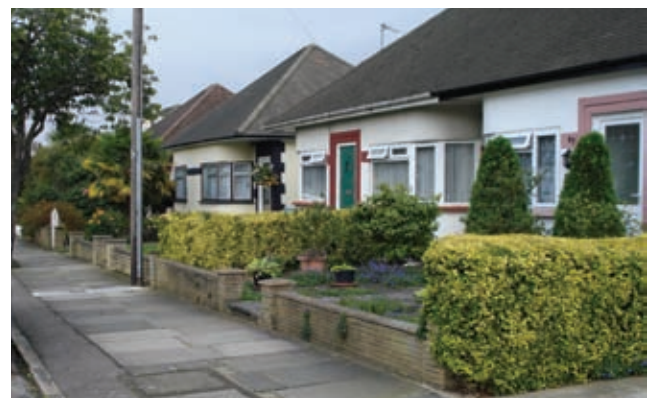
6. Original details – low stone boundary wall with piers and roof tiles.
