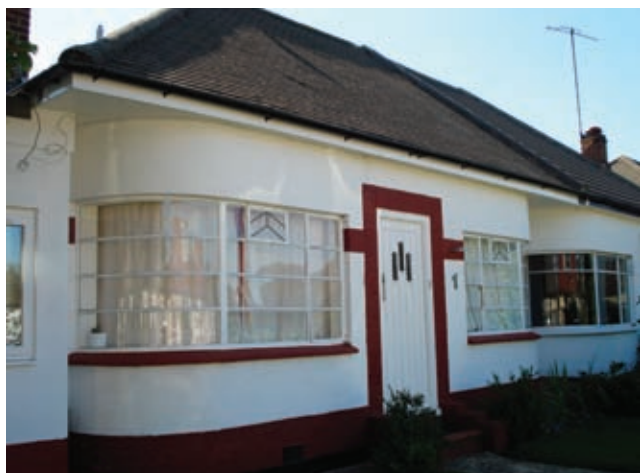
1. Original details – fenestration, door with glazed panels, brick bands (although painted over), roof tiles.
