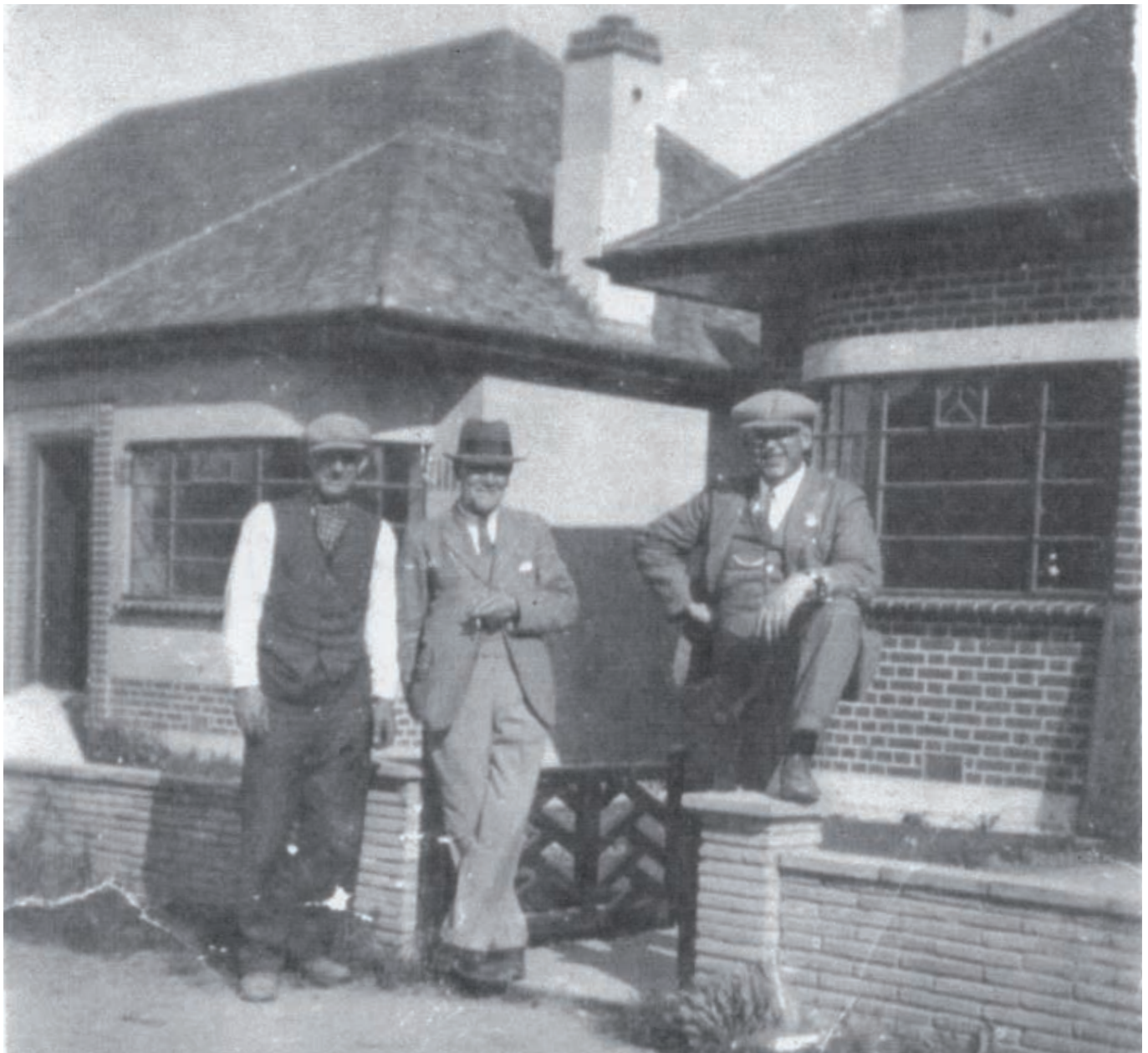
39 and 41 Gladstone Avenue, when newly built in 1937. Note the original detailing: low stone boundary wall with gate piers and timber gate; roofscape, roof covering and chimney stacks; metal windows with curved profile. Source: Stephen C. Randall.
