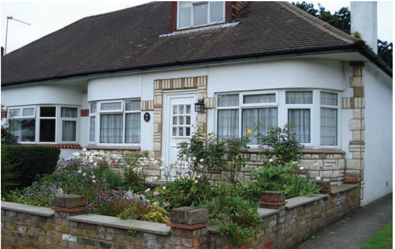
3. Original details – front garden planted, roof tiles. Inappropriate alterations – front dormer, brick cladding, fenestration, chimney truncated.
