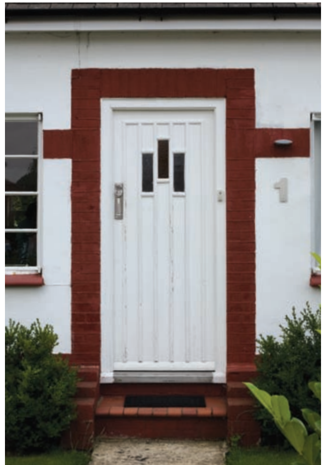
10. Original detail – original door
