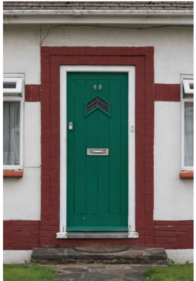
8. Original detail – original door
