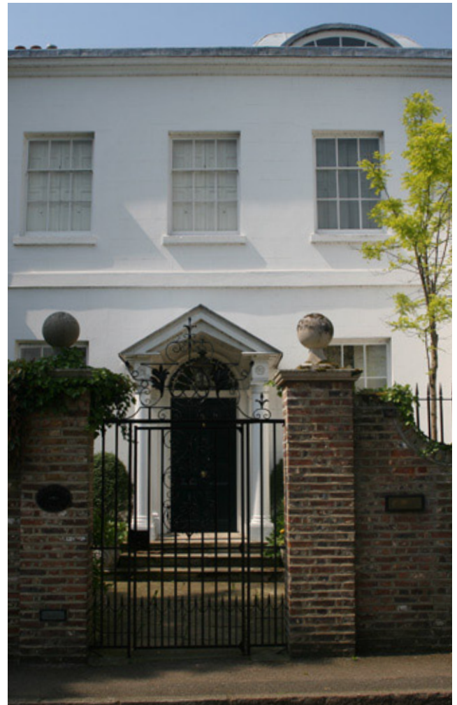
Petersham Lodge, River Lane
