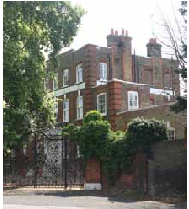
Typical mansion set back from Petersham Road
