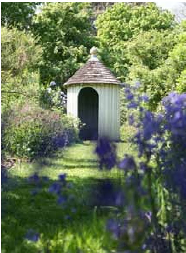
Garden building, Ham House Gardens
