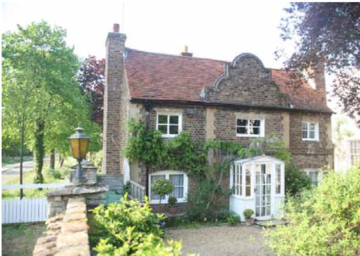
Great South Avenue and C17 brick lodge with distinctive gable
