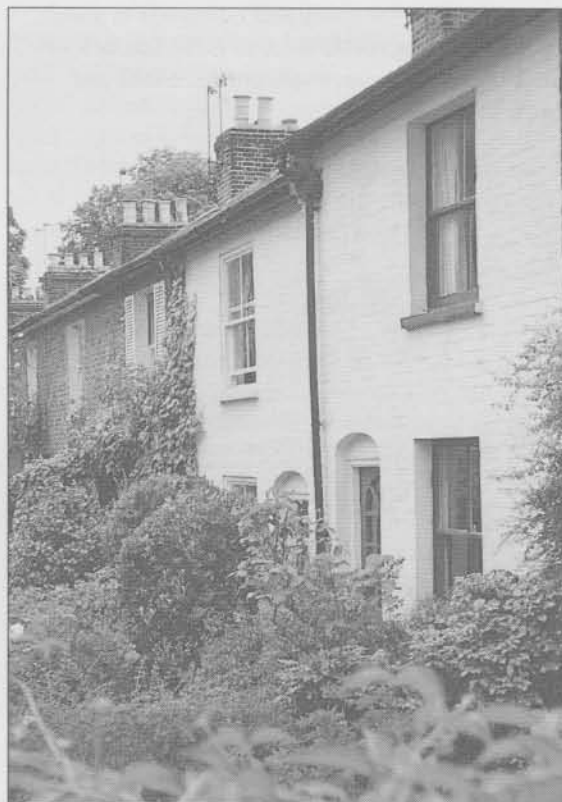
View along nos. 1-13 Park Cottages
