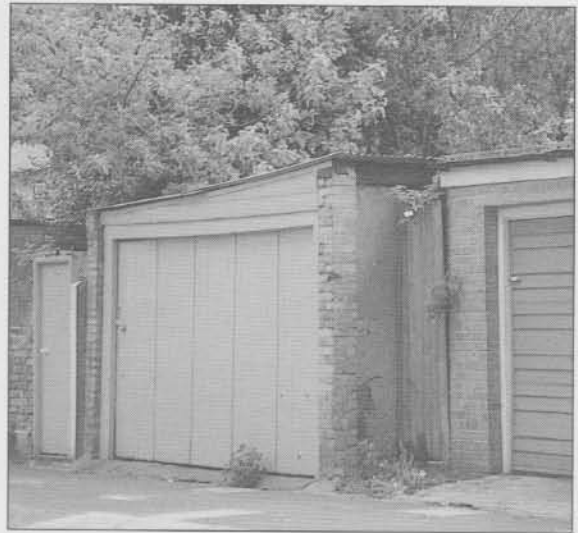
Unsightly garages facing onto Rosslyn Road
