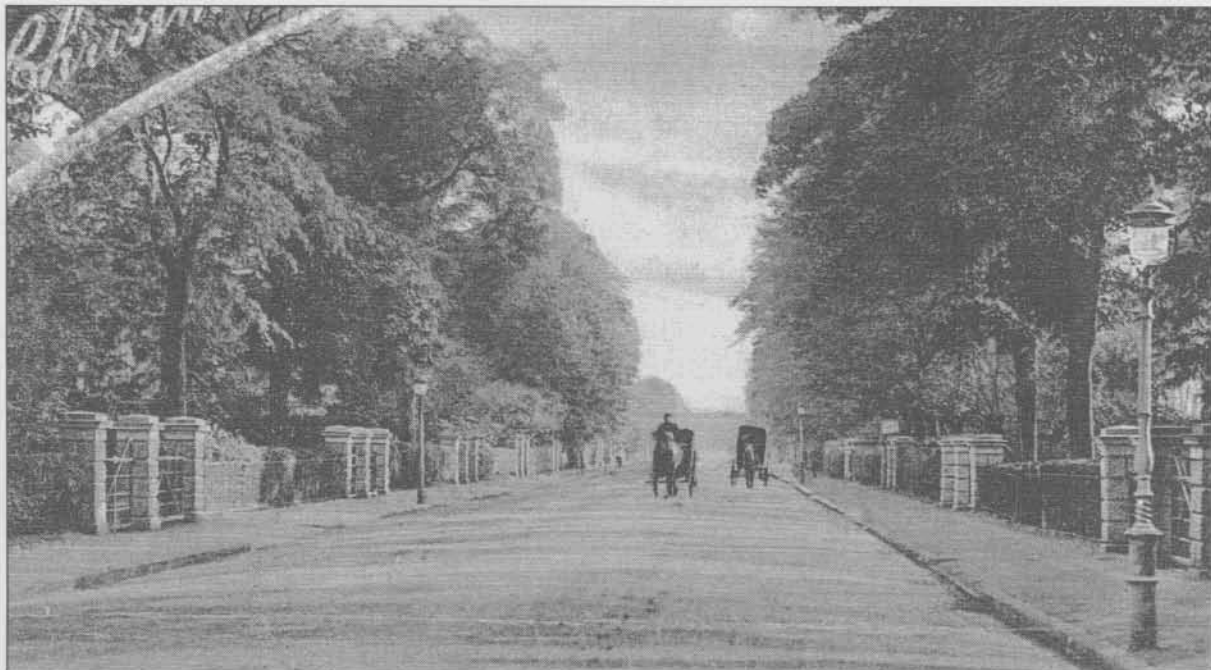
Castelnau at the beginning of the C20th
