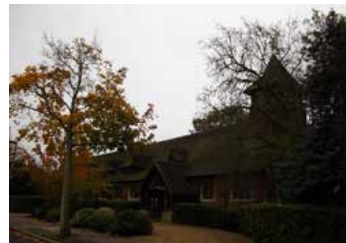
Barn Church, Atwood Avenue
