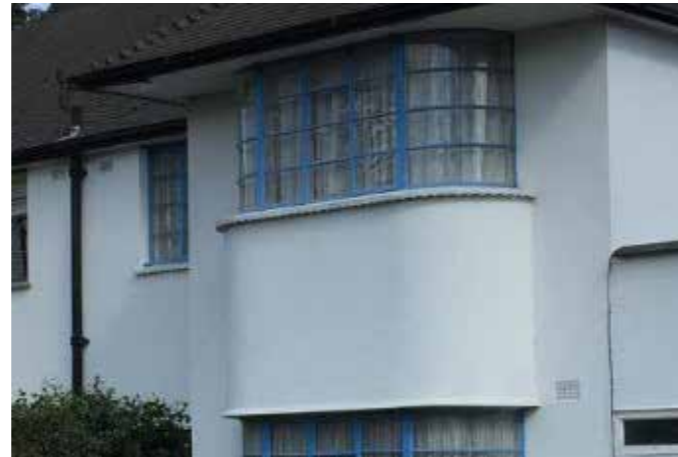
Critall-style casement steel window in an interwar house
