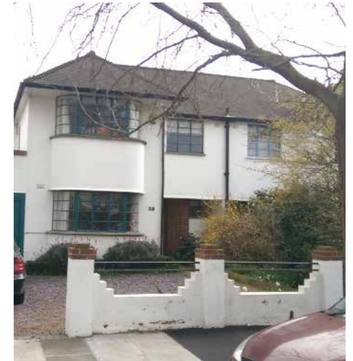
Boundary wall, Beresford Avenue
