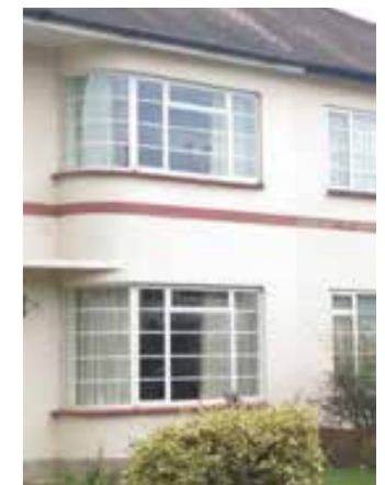
Critall-style casement steel window in an interwar house
