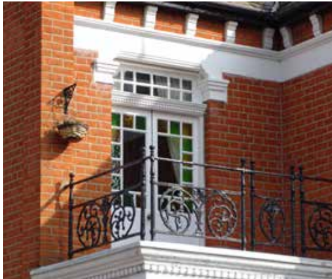
Timber casement balcony doors with Iron railing balustrade
