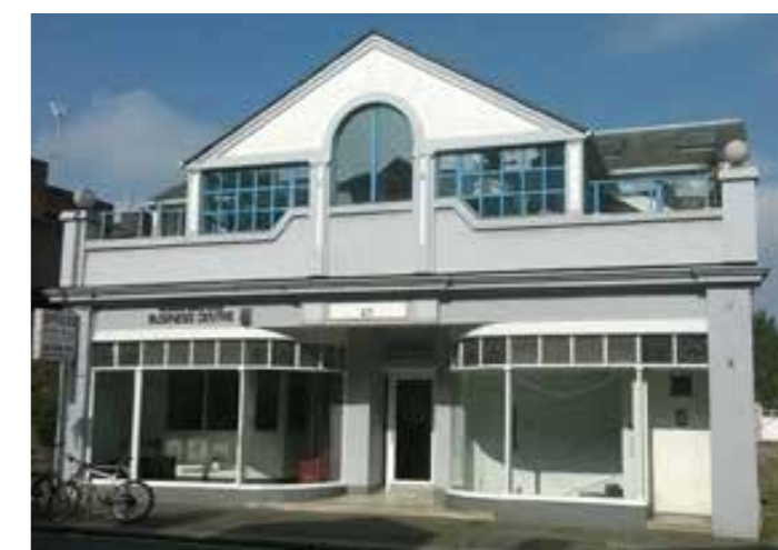
No. 419 Richmond Road - Art Deco Commercial unit
