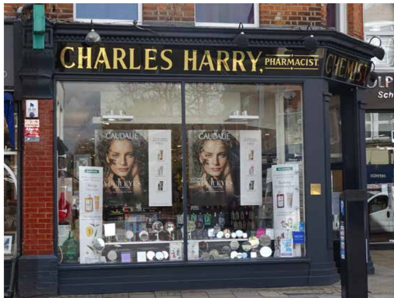
A good example of a reverse painted gilded glass fascia, set at an incline with a dentiled cornice. Large plate glass shopfront with surviving glazed tiled pilasters with console brackets
