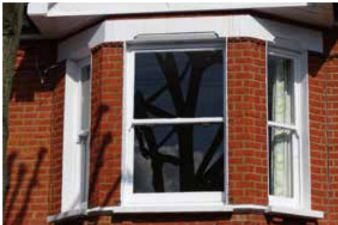
Timber sash window in a c. 1900 house
