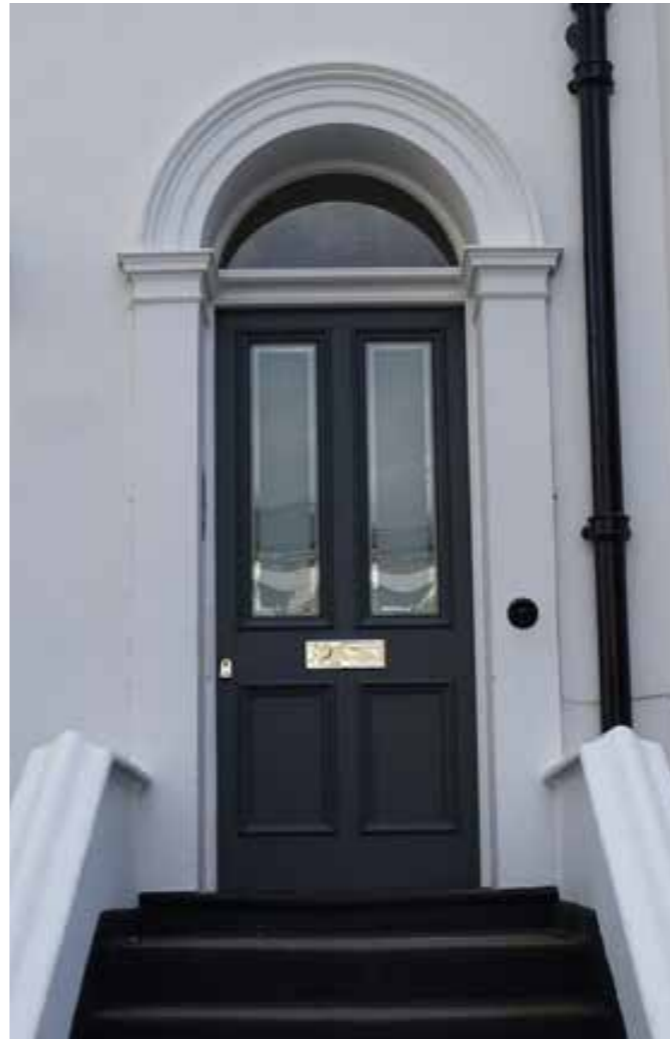
Timber panelled double doors with curve fanlight
