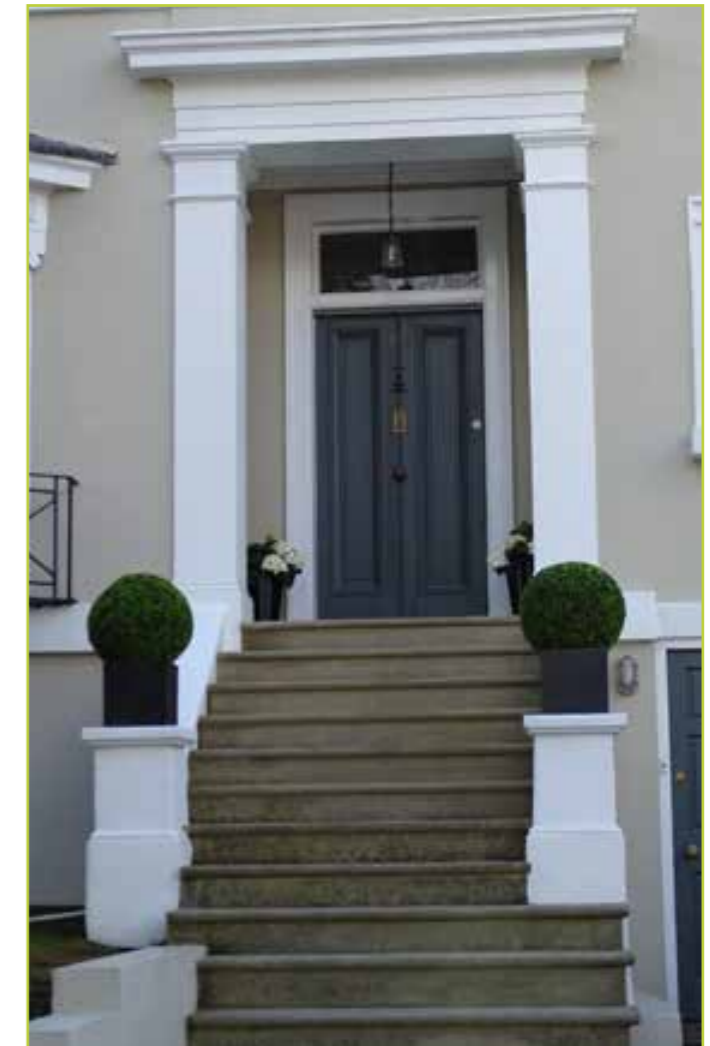
Georgian doorway with simple white painted columns and lintel framing the entrance
