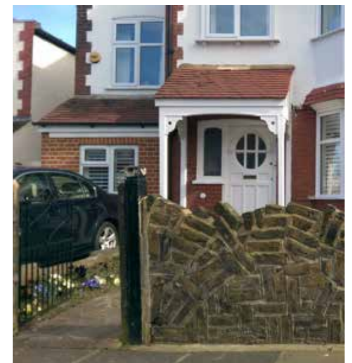
Boundary wall, Clydesdale Gardens
