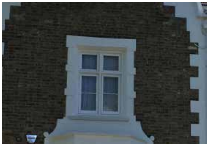
Timber casement with mullion and Queen Anne style transom in a Victorian house
