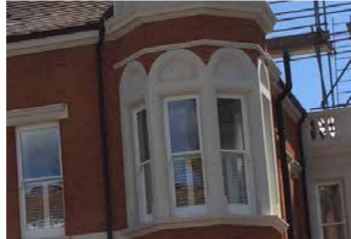
Timber sashes in a Victorian turret
