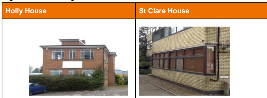
Figure 3.23 Existing offices at St Clare Business Park
