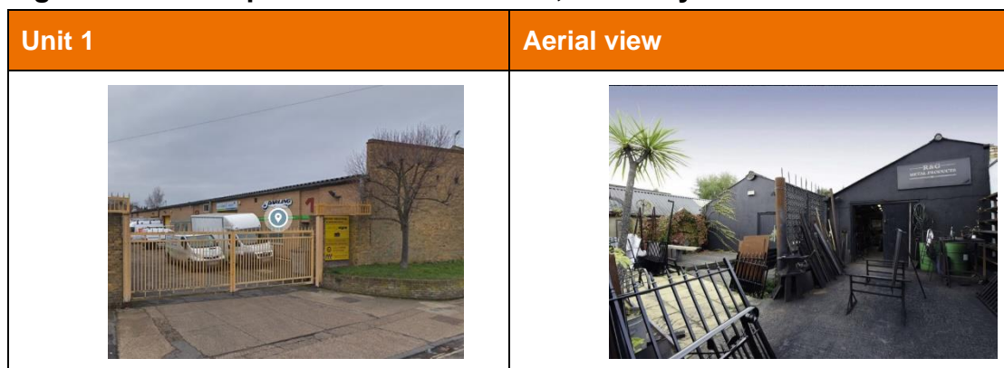
Figure 3.10 Examples of industrial units, Mereway Road Industrial Estate
