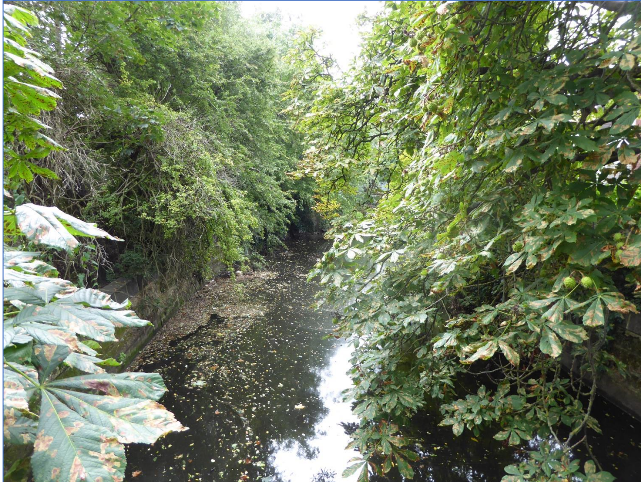
Figure 53: River Crane showing concrete channel
