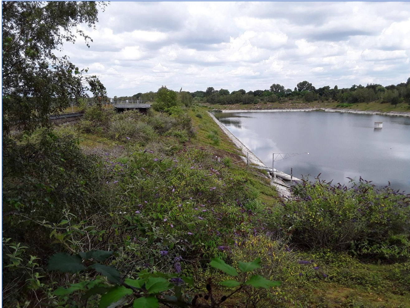
Figure 26: Vegetated reservoir walls at Stain Hill reservoir
