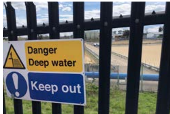
View from outside General Area on northern boundary towards south
