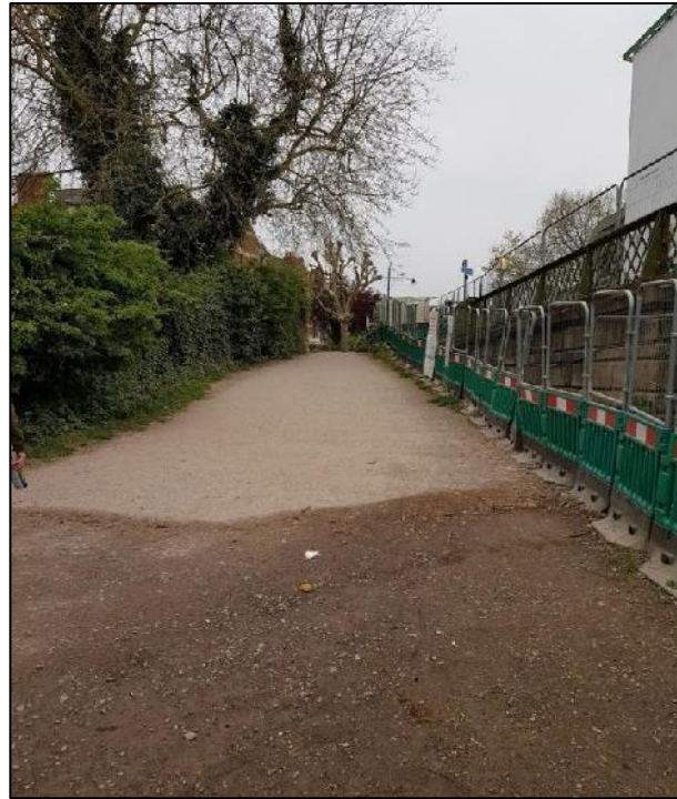
Figure 2-3: Concrete Path to the Side of Hammersmith Bridge
