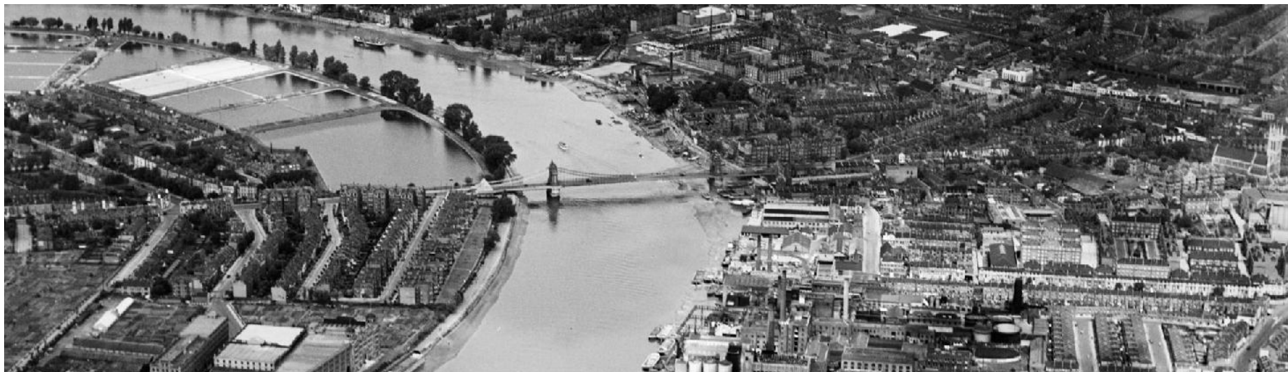
Fig. 13: Aerial view of Hammersmith and Castelnau, 1938
