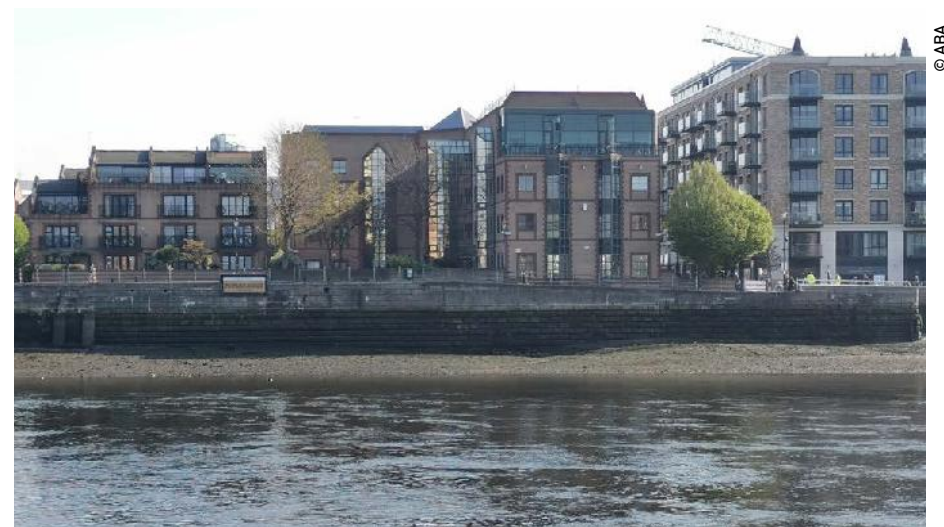
Fig. 36: Locally listed river wall, viewed from the southern Thames Path
