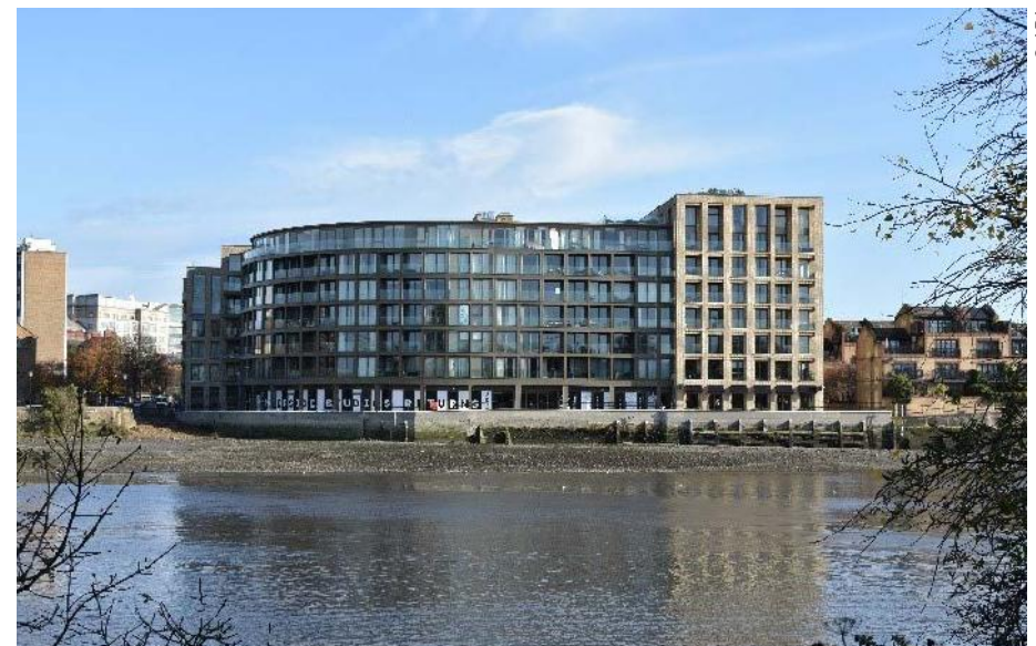
Fig. 15: Riverside Studios residential development, 2020
