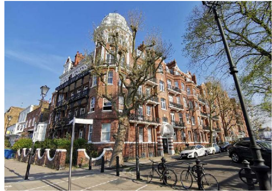
Fig. 31: Digby Mansions, viewed from the northern Thames Path
