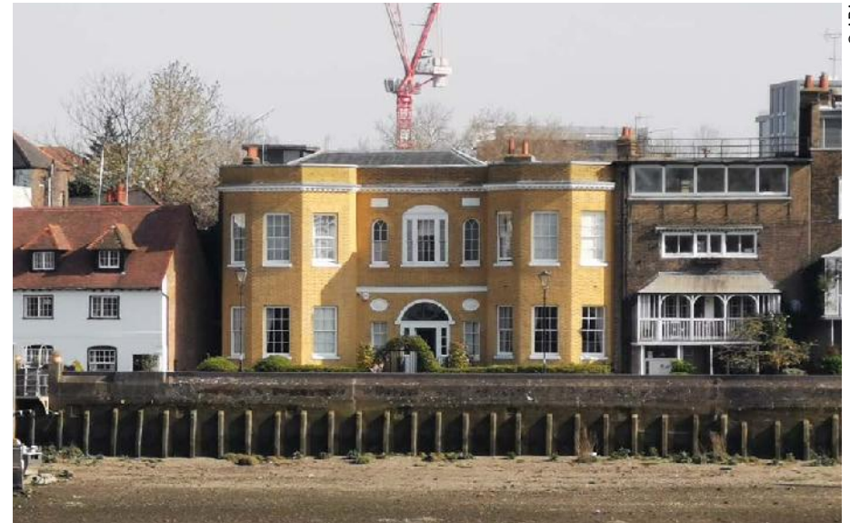
Fig. 22: No. 10 Lower Mall (Kent House)
