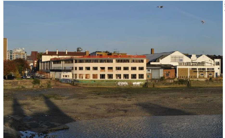
Fig. 14: Queens Wharf and Riverside Studios prior to demolition, 2014
