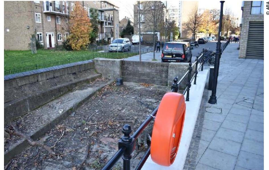
Fig. 35: Locally listed drawdock adjacent to the bridge
