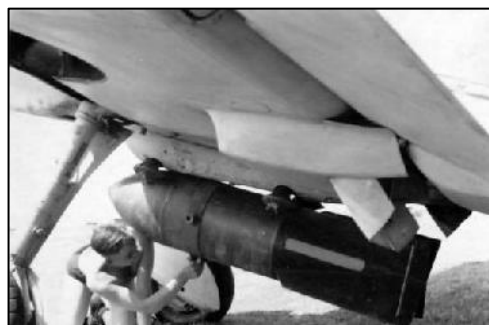
SC250 attached to undercarriage of Messerschmitt Bf109
