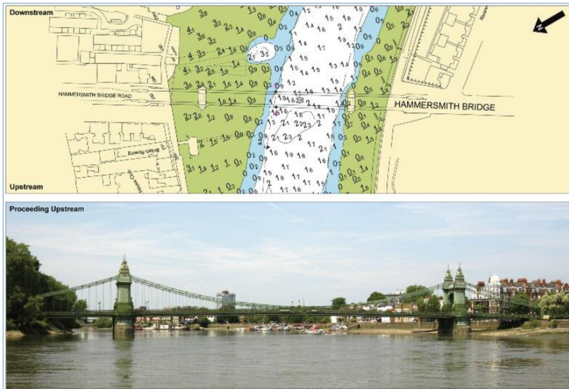
Figure 1: Extract from PLA Guide to Bridges 2012 showing Hammersmith Bridge.
