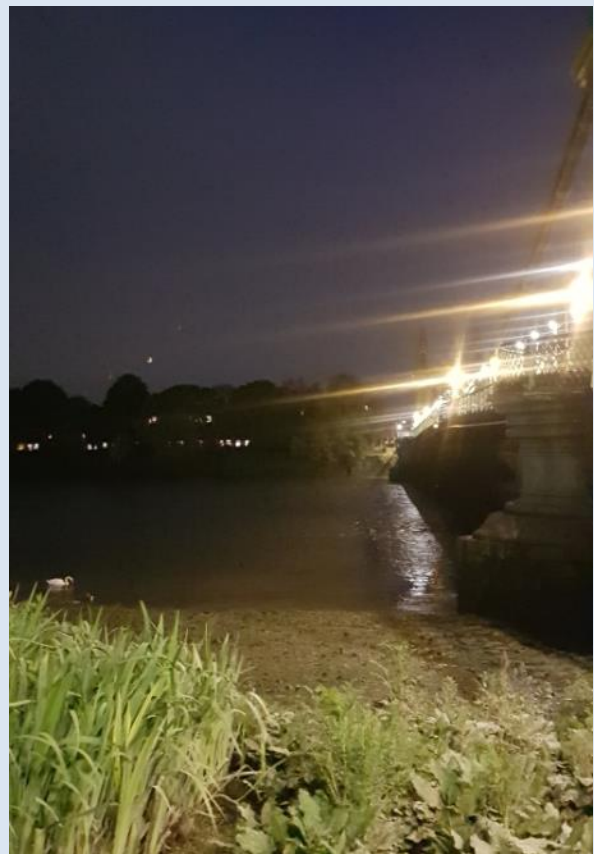
Light spill alongside the northern bridge abutments (taken August 2020)
