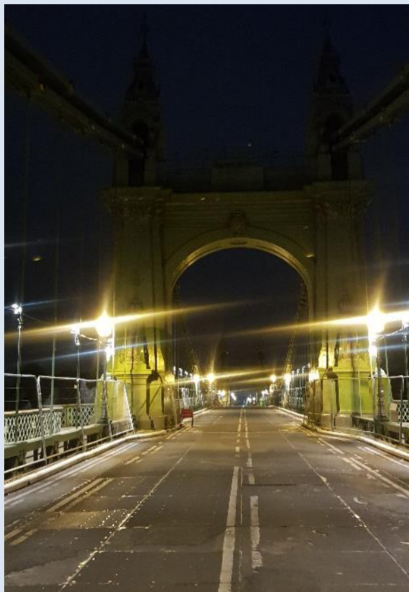
Light spill along the existing Hammersmith bridge carriageway (taken August 2020)
