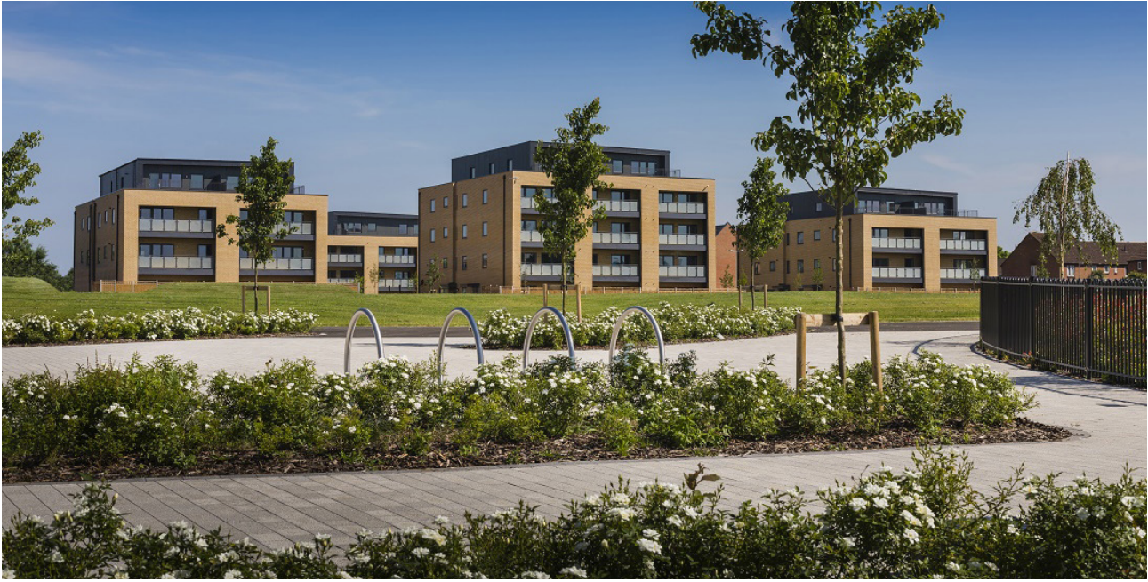
Fountains Close, RHP. Provides a mix of affordable rent and shared ownership
