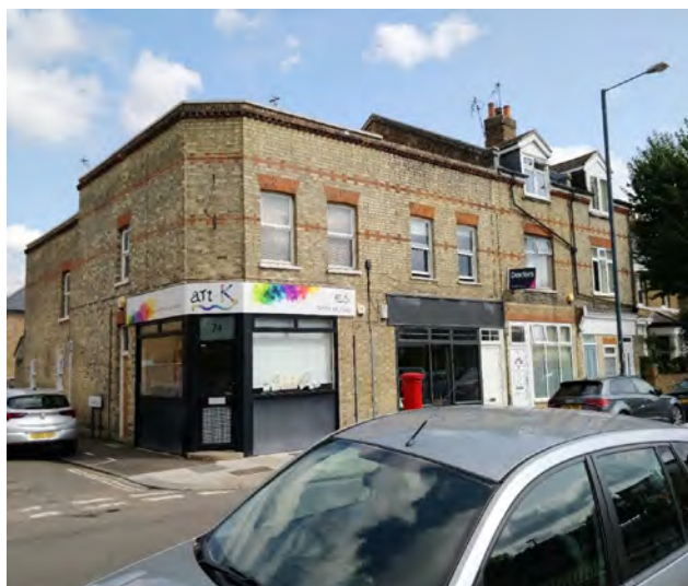
No.s 68-74 Abercorn Road; evidence of former shopfronts with only 74 remaining.
