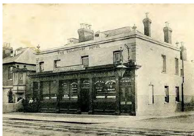
Willoughby Hotel, 59 Church Road, bombed in November 1940 (Source: https://pubshistory.com/Middlesex/Teddington/WilloughbyHotel.shtml ).
