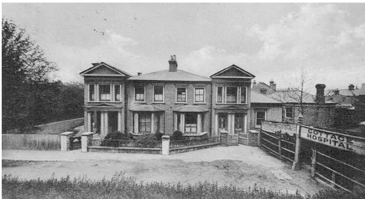
The Teddington and Hampton Wick Cottage Hospital, established in 1875, with dispensary behind, built in 1883. (Source: Richmond Local Studies Archive)
