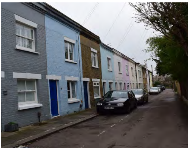
Row of colourful cottages in School House Lane.
