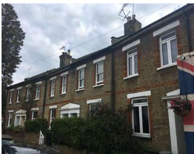
Houses with pedimented porches and double entrances in Wick Road.
