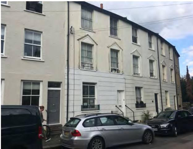
Curved terrace in Wick Road.
