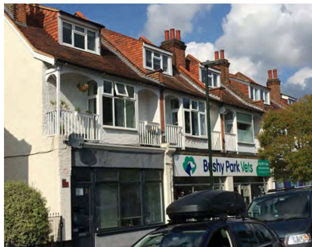
Shopping parade with timber balcony detailing in corner of Bushy Park and Kingston Roads.
