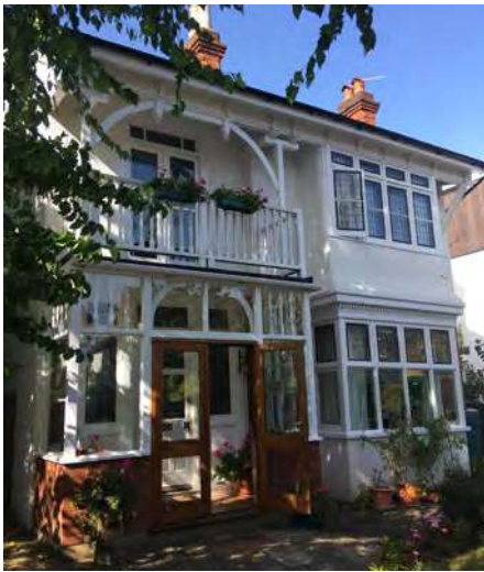
Decorative timber entrance porch with verandah above.
