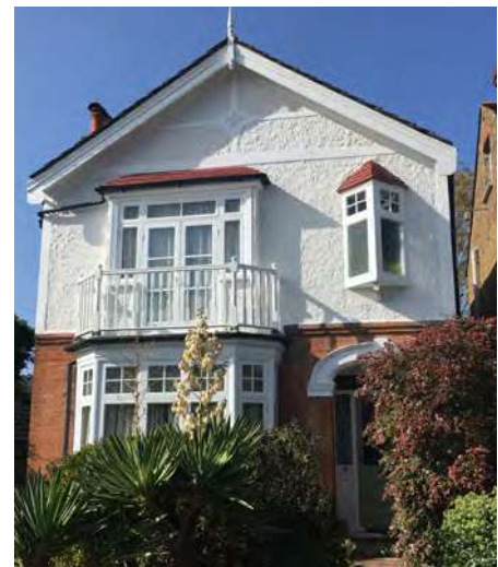
Detached house with bay window and balcony above, inset porch, oriel window and gable detail.
