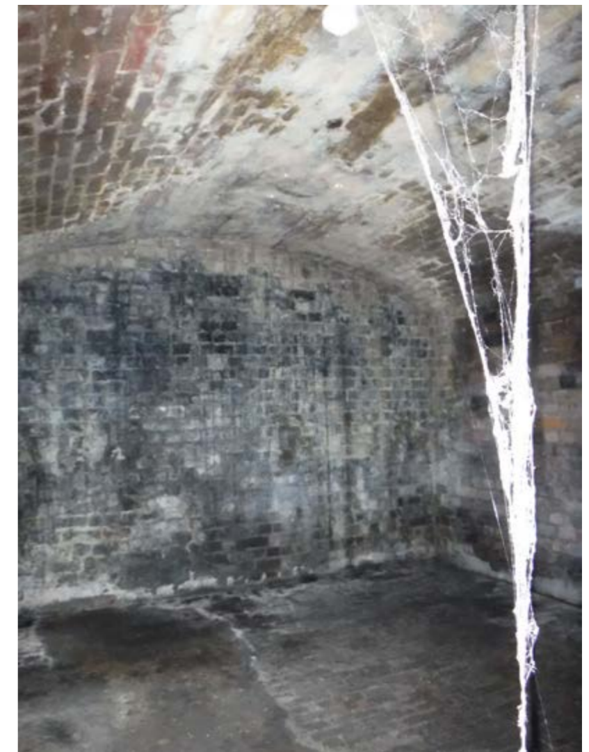
Figure 57: Damp basement
