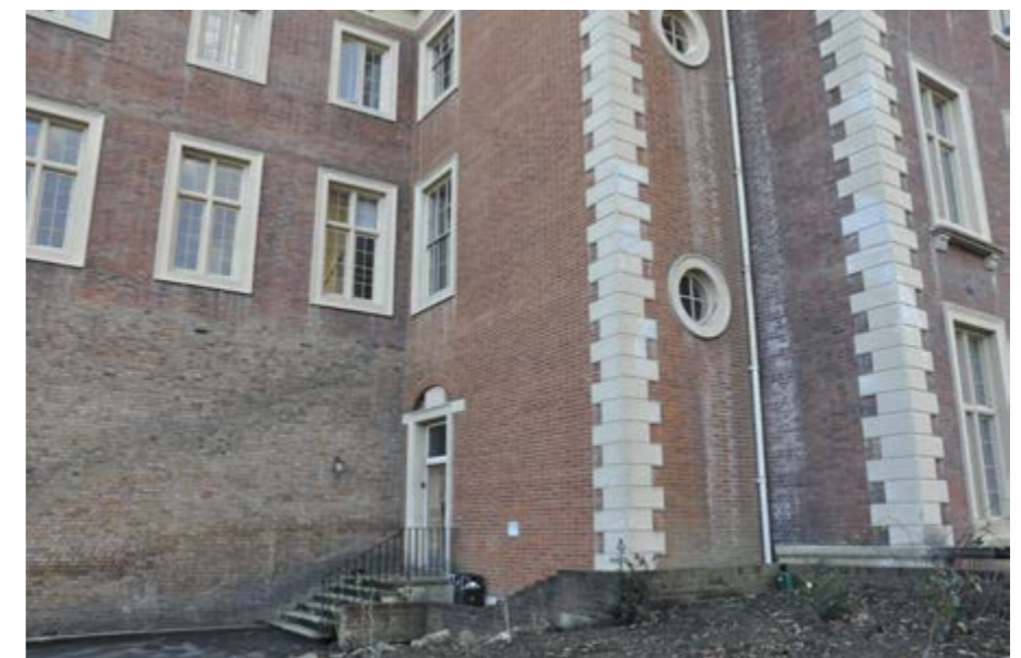
Figure 39: Exterior of 1970s staircase extension
