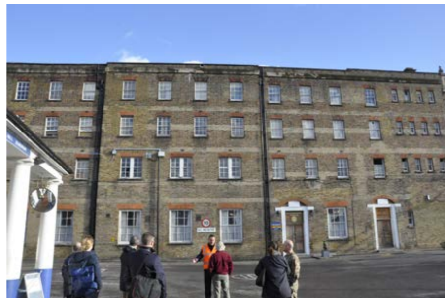
Figure 38: Western elevation of west wing
