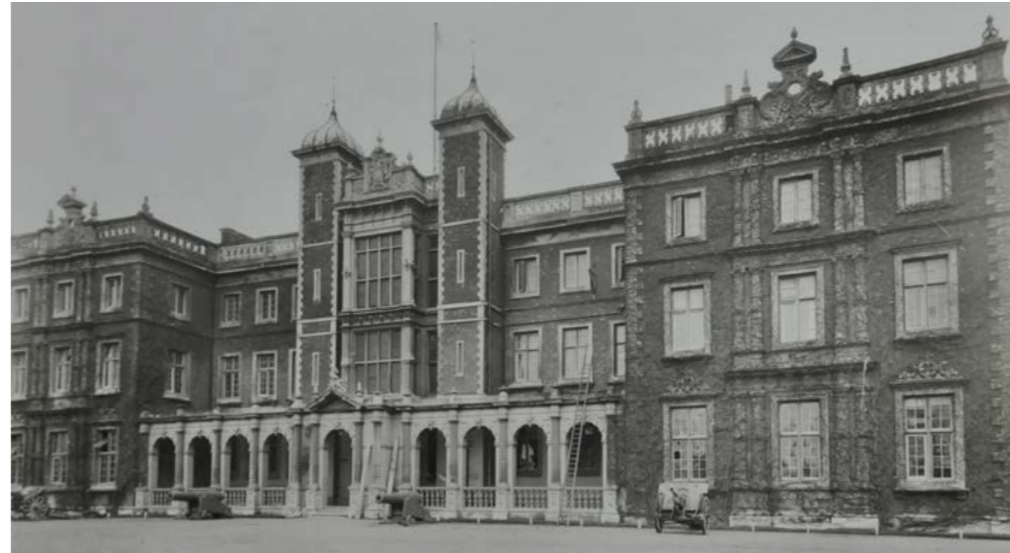
Figure 17: Front elevation as captured by the stonework inspector in 1921
