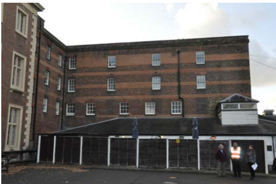
Figure 37: View of northwest wing from the east, showing the patched brickwork and the subsidiary building in front
