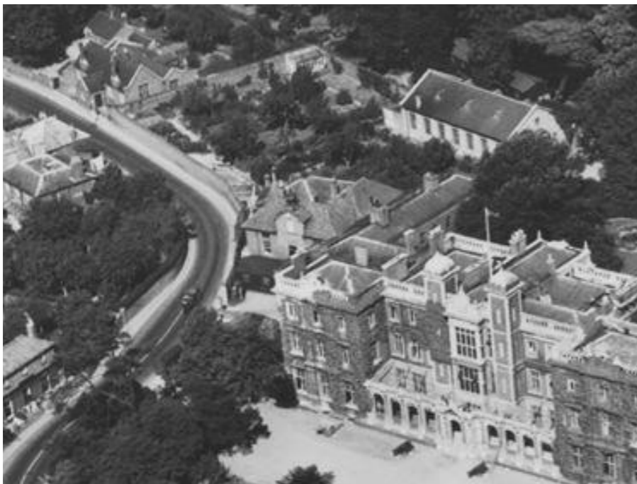
Figure 20: Aerial view from c.1930s showing the front elevation of the guardroom more closely resembling that of 1711. The former band practice room can be seen behind
