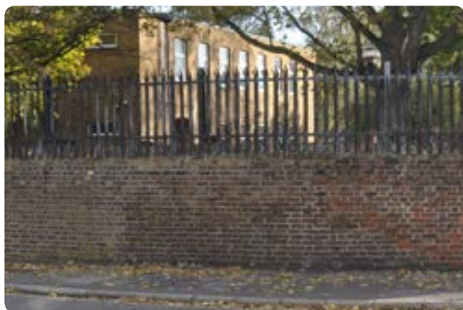
Brick wall with palisade fencing
