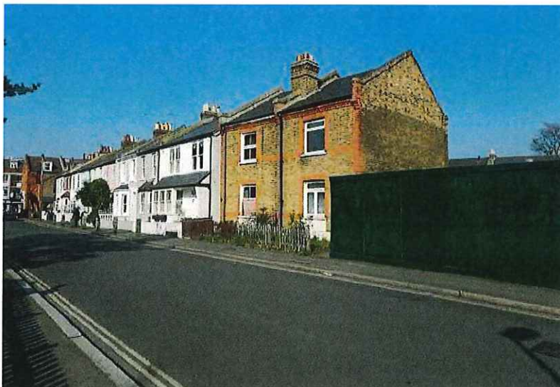
North Lane Depot from North Lane
