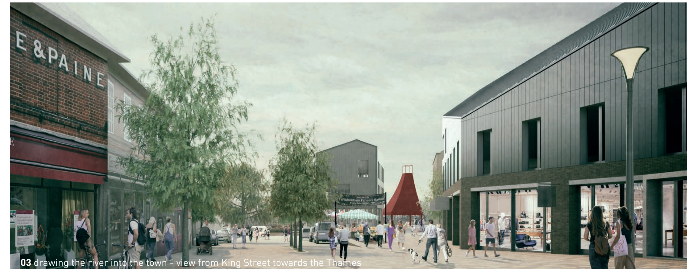
03 drawing the river into the town - view from King Street towards the Thames
