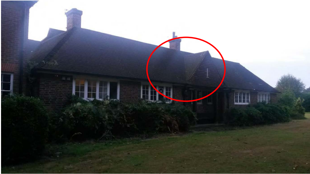
Photo 1 – Soprano pipistrelle emerges from western side of building from location shown
