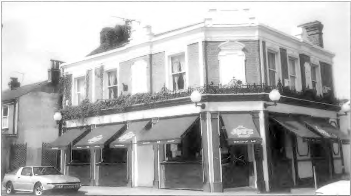
No. 99 (Joe's PH): Good quality feature brickwork and stucco mouldings to first floor. Decorative ironwork above cornice
