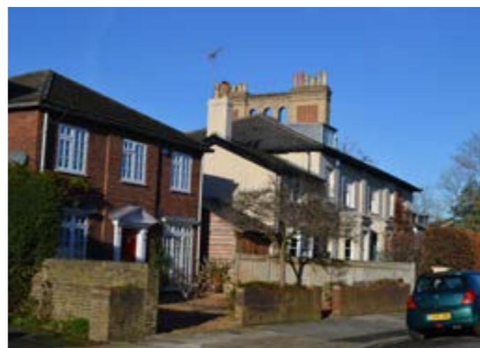
View north along Pope's Avenue
