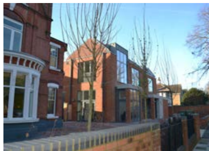
Newland House School
