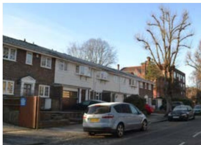
Small row of terraced housing at east of Waldegrave Park
