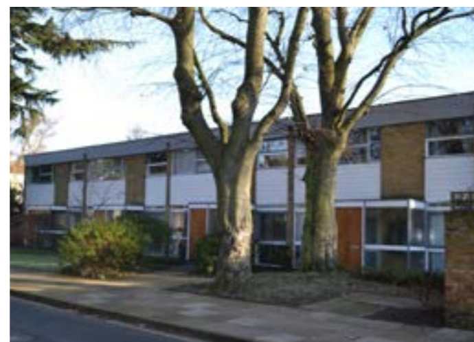
Two storey uniform terraced housing
