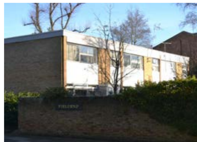
The houses are built of stock brick and have two-tone painted timber windows
