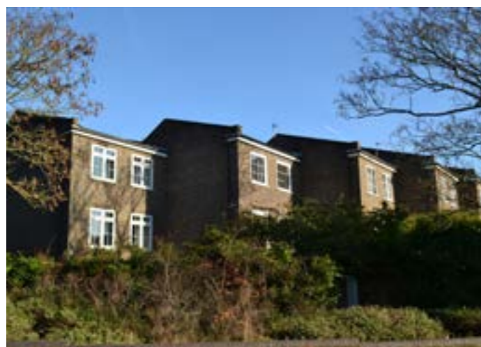
Back of Fortescue Park
