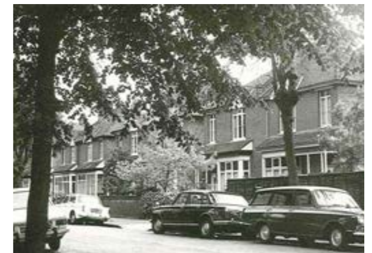
1973 photograph of 22-24 Walpole Road
