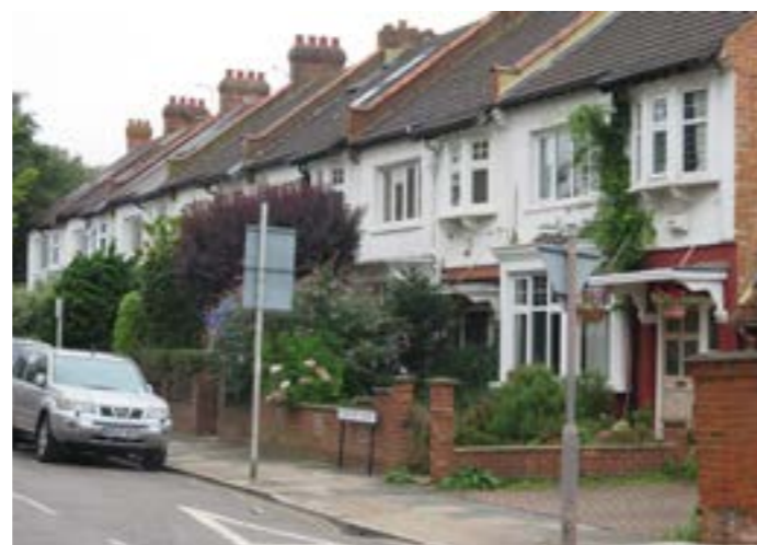
Radnor Road looking north
