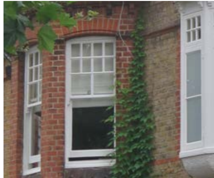
Double hung sash windows
