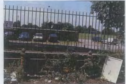
Fig.103 In front of the Royal Hospital the old RB cast iron bollards mark where the clairevoie allowed views into the Park
