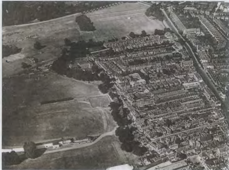
Fig.101 1940s Aerial showing the open flow of the parkland between the Cricket and Athletic Grounds and the golf course. Note the Royal Laundry amongst mature trees
