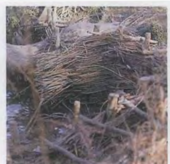
Fig.112 Willow spilling could be used to re-instate the river edge in further places
