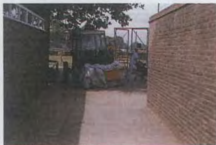
Fig.88 Maintenance equipment blocks the narrow and obscured entrance to the playground in the south park
