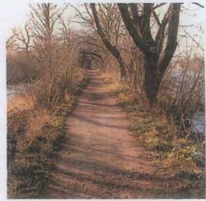
Fig.47 The towpath runs on a kind of raised causeway which was built out into the river in 1766/72, creating an internal ditch separated from the main watercourse of the Thames
