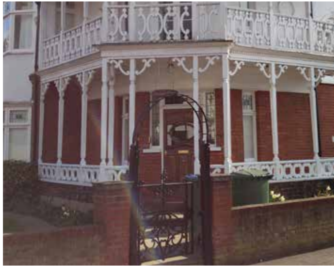
Ornate white painted wooden porch and canopy entrance with original painted door in a stained glass surround
