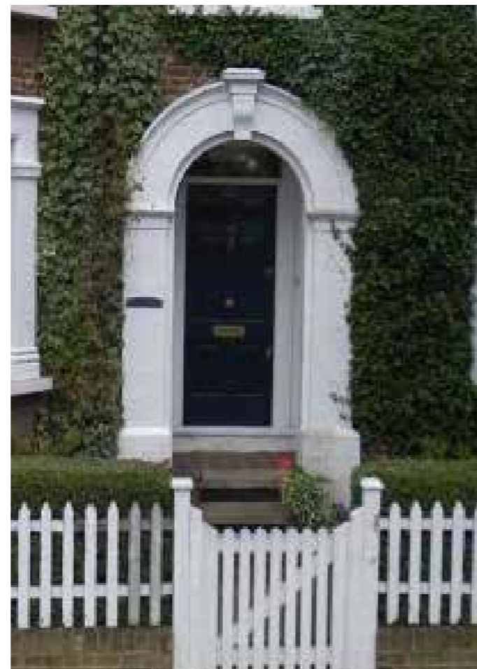
Timber door with fanlight above and a classical white painted curved entrance
