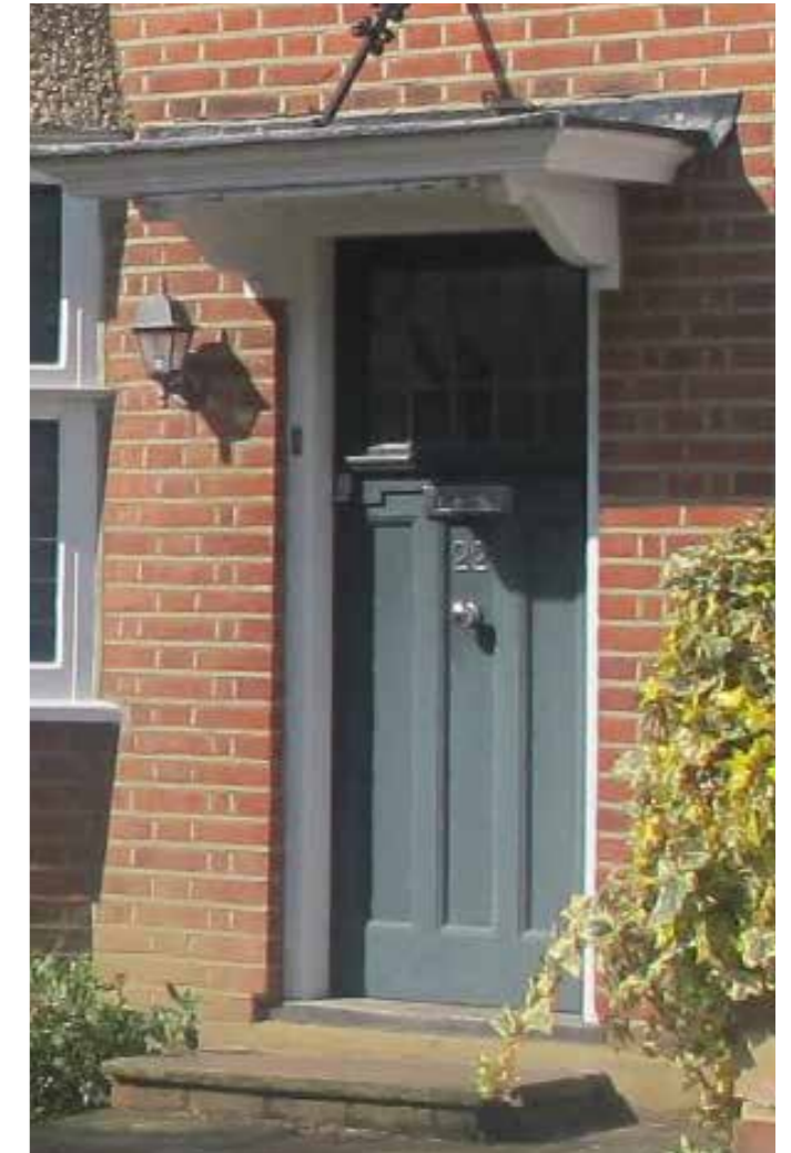
Original painted door, flat roof canopy and white painted cornices
