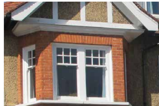
Sash windows with hybrid design set in the canted bay of an interwar property
