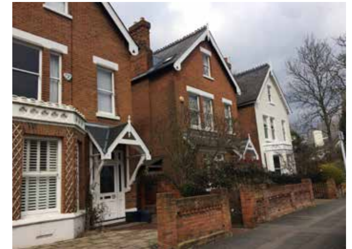
Boundary walls, Seymour Road
