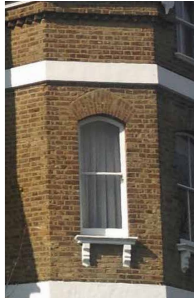
Victorian property with narrow sash windows curved with the aligning brickwork. White quoining above and below
