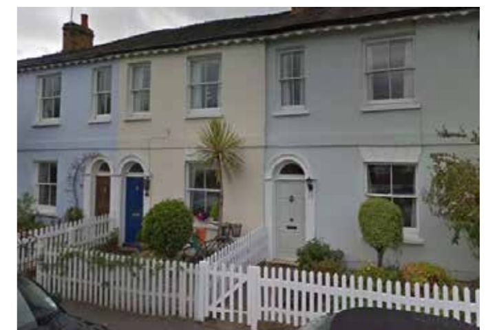
Station Road, White picket fencing
