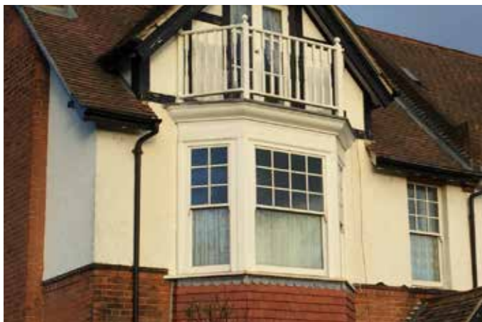
Timber sash window, partially Criticalled, with timber Balastrade atop
