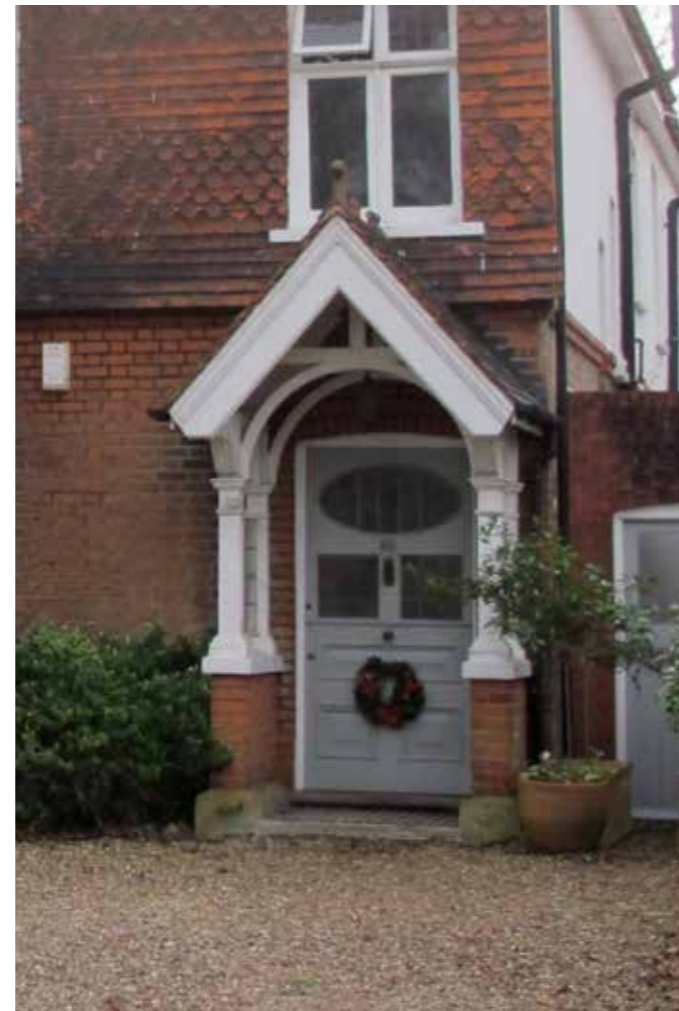
Timbercase door with distinct glazing and curved fanlight atop. The entrance is framed by an ornate gable fronted porch.
