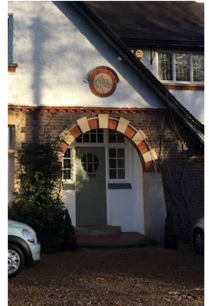
Edwardian property with curved recessed entrance in render and brick, ornate date stone.
