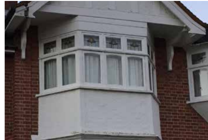
Canted bay windows with original stained glass work on an interwar house
