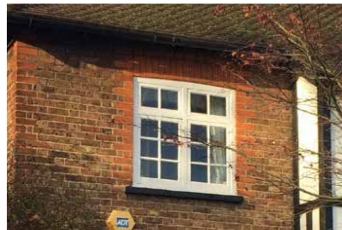
Timber casement window in a Late Victorian house
