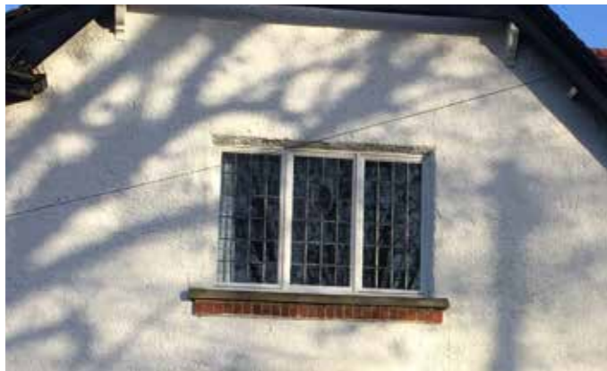
Critical windows with timber casements and bricked window ledge
