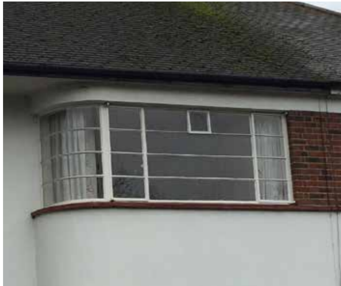
Art deco style curved metal framed window
