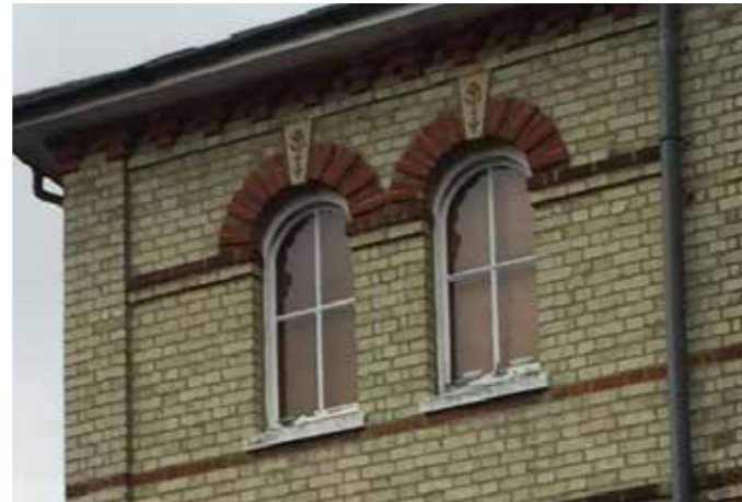
Curved sash windows with stock brick keystone
