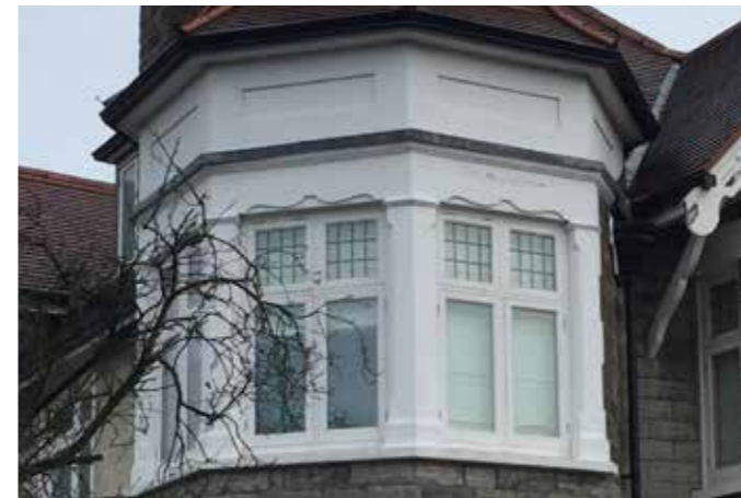
Timber casement window in a Victorian house
