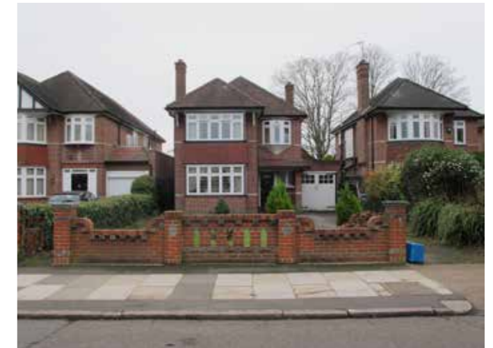
St James's Road, Boundary Wall
