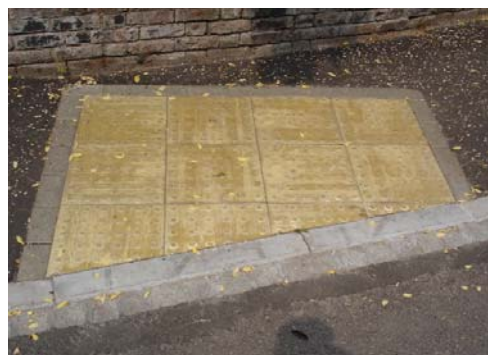
Tactile paving with brick surrounds
