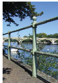
Ranelagh Drive railings
