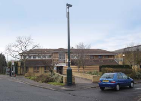
Intrusive siting of CCTV
