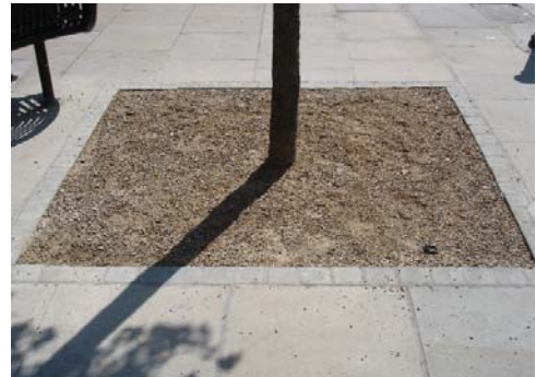
Breedon gravel tree surround
