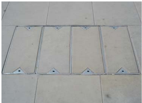
Neatly finished manhole cover
