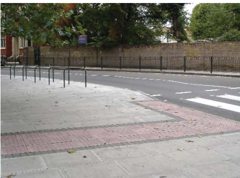
Avoid long tails on tactile paving
